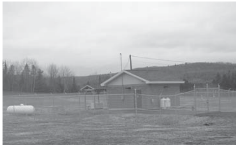
New Groundwater Plant
