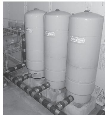
*Example of Pressure Tanks: Note only one pipe serves as both inlet and outlet, no separate outlet*
