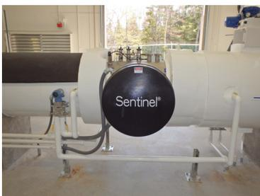
Bangor Water District started their project in 2011 with 2012 DWSRF funds and a preliminary design by Black & Veatch. Construction began in 2013 with T. Buck Construction, using 2013 DWSRF funds on a new UV building to house two Sentinel
