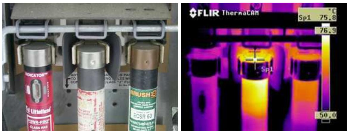
Figure 26: Overheating fuse (Courtesy of FLIR Systems, Inc., N. Billerica, MA)
