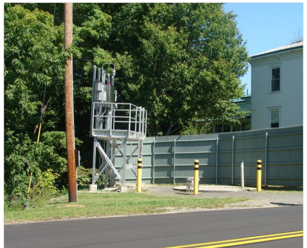
The pump station on Elm Street was replaced in 2007, followed by improvements to sewer pipes serving area residences in 2009.
