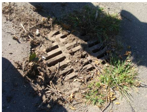
Stormwater catch basins require regular maintenance in order to remain clean and clear of debris, trash, and sediment.
