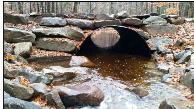
After: Beaver Brook, ten-foot culvert
