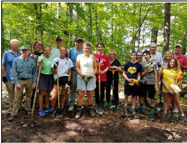
Volunteers participated in a hands-on workshop installing conservation practices for a residential property.
