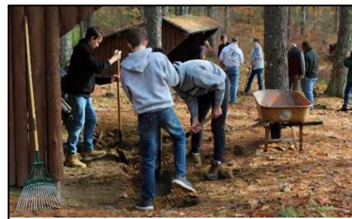
Boy Scout Troop 73 installed roof dripline trenches at Camp Hinds lean-tos.
