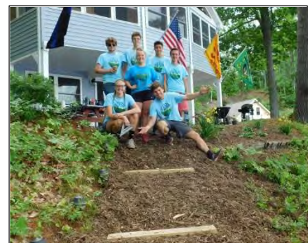
AWWA's YCC installed 58 BMPs on eight properties on Great East Lake.
