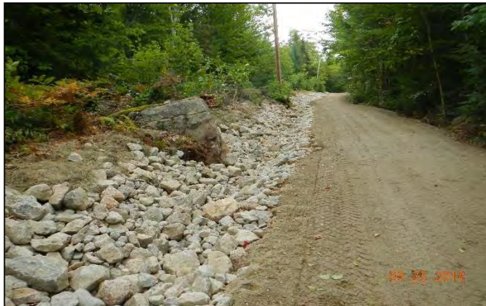
Riprap-lined ditches and other road BMPs were installed through the project.
