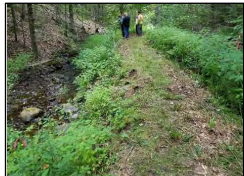
Prior to work on one project site on the lower reach of Tributary C, there was significant stream channel incision and erosion adjacent to walking trail-sewer line.
