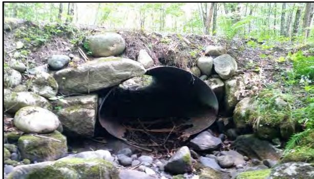
Before: Beaver Brook, four-foot culvert
