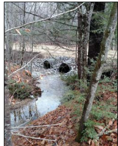
This road crossing of a Crooked River tributary had washed out due to an undersized culvert. The 24” culvert was replaced with both a 48” culvert and a 36” overflow culvert.
