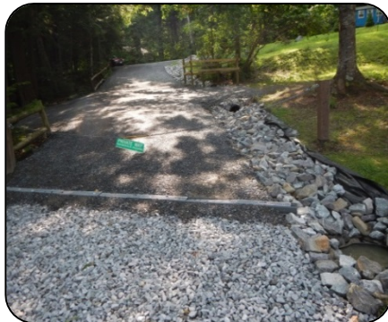
Project partners and work completed (left to right): local road association volunteers install BMPs at boat launch; volunteer retired road expert checks a newly installed culvert and plunge pool; boat launch newly stabilized and with runoff diverters, culverts, plunge pools and rock-lined ditches; and YCC members at a work site.
