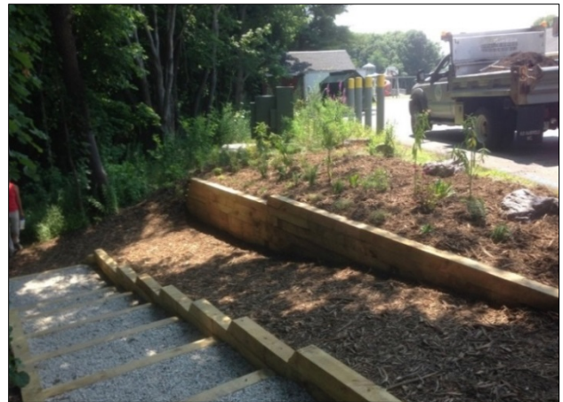
Infiltration steps, buffer, and erosion control mulch installed behind the Kittery Community Center.
