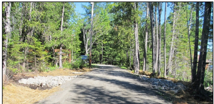
Rock cannolis used to pass water from a wooded wetland to the lake and stabilize the camp road.
