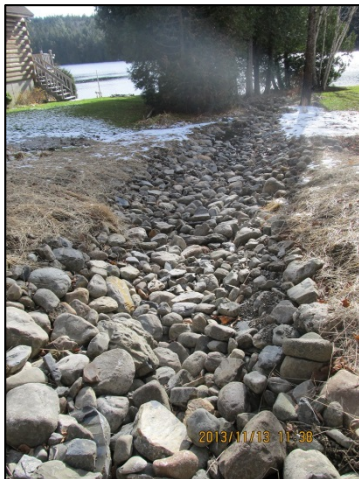
Stabilized cross-culvert outlet and ditch to a buffer.
