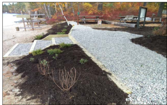
After - Volunteers spread erosion control mulch, planted native vegetation, and installed water bars to help manage runoff and stabilize eroding areas.
