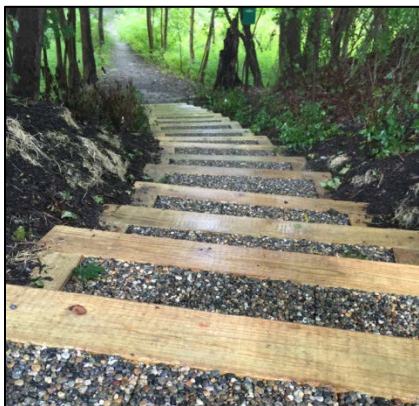
Infiltration steps installed to treat runoff and stabilize an eroding trail leading to Trout Brook.
