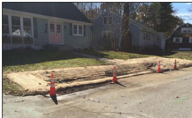
A rain garden was installed on Simmons Road in partnership between the City of South Portland and the adjacent homeowner.
