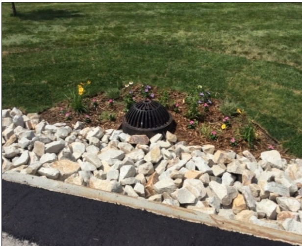
Biofiltration system installed along a roadway.
