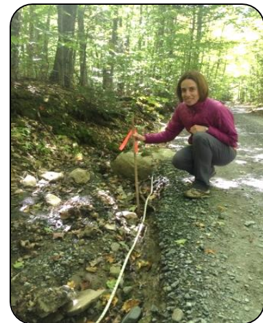
A gravel road ditch eroding sediment and phosphorus into Parker Pond.
