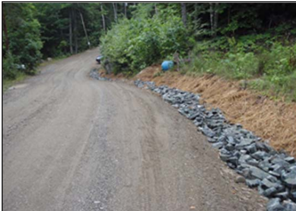
Gravel road stabilized by crowning its surface & installing a road ditch with turnouts
