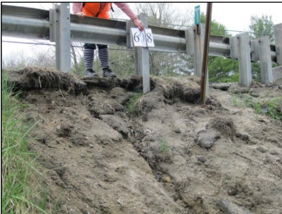
Erosion at road embankment
