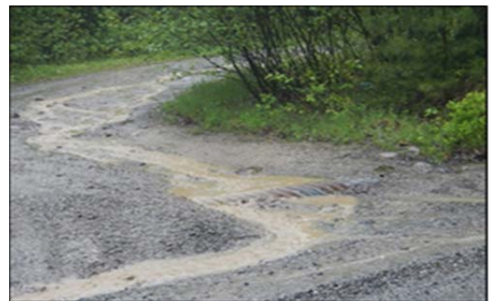
Sediment from eroding gravel camp roads carried in runoff to the lake
