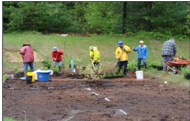
Volunteers adding plants to subsurface bioretention cell at the Russell Road Conservation Area
