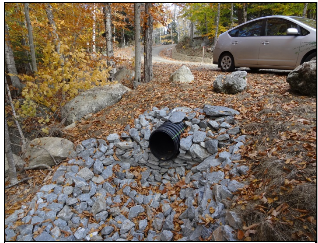
Rock-lined culvert outlet on unpaved camp road
