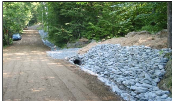
Rock-lined road ditches prevents erosion, keeps sediment from reaching lake
