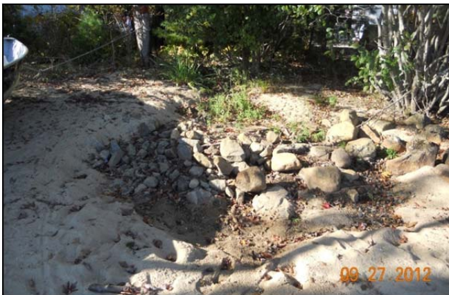
Before: Eroded area, sediment entering lake
