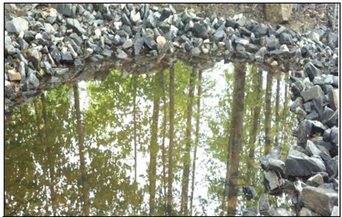
After: Settling basin installed to trap sediment
