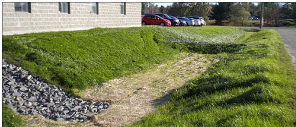
Soil media filters help cool water, trap pollutants, and slow the flow of runoff into Blanchette Brook
