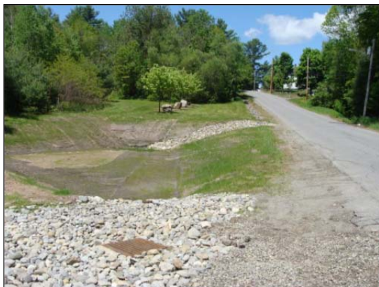
Subsurface bioretention cell to treat stormwater runoff
