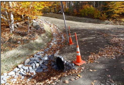
BMPs installed on gravel roads
