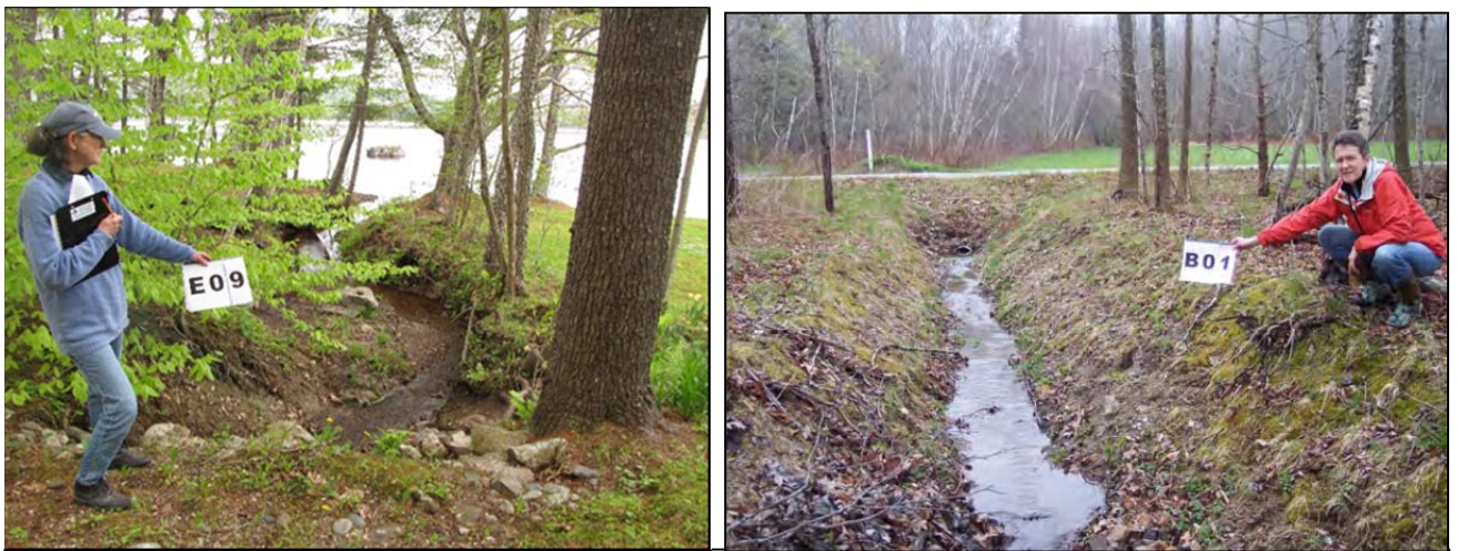
Volunteers document erosion and sediment problems in the Alamoosook Lake watershed
