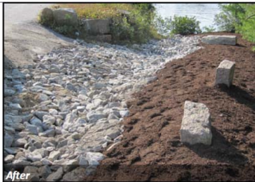
This heavily eroded access site on the Route 302 causeway in Bridgton was stabilized using stone riprap and erosion control mulch. Key goals of protecting water quality include diverting, spreading out, and infiltrating runoff.
