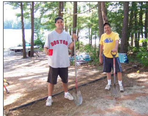
Landowners install a rubber razor to divert driveway runoff into a buffer.
