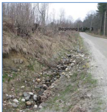
Before – eroding bank and ditch
