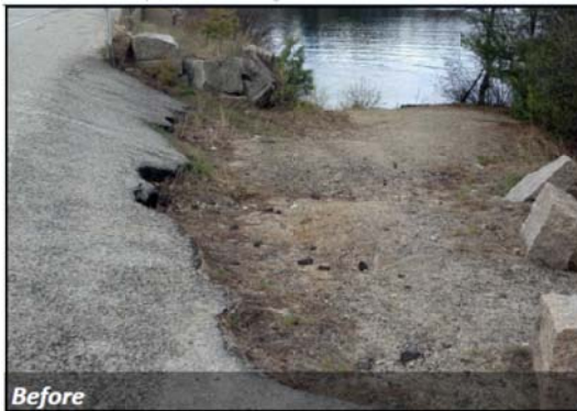
This heavily eroded access site on the Route 302 causeway in Bridgton was stabilized using stone riprap and erosion control mulch. Key goals of protecting water quality include diverting, spreading out, and infiltrating runoff.
