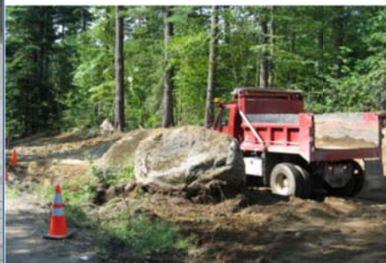
During – removing bank, including large boulders
