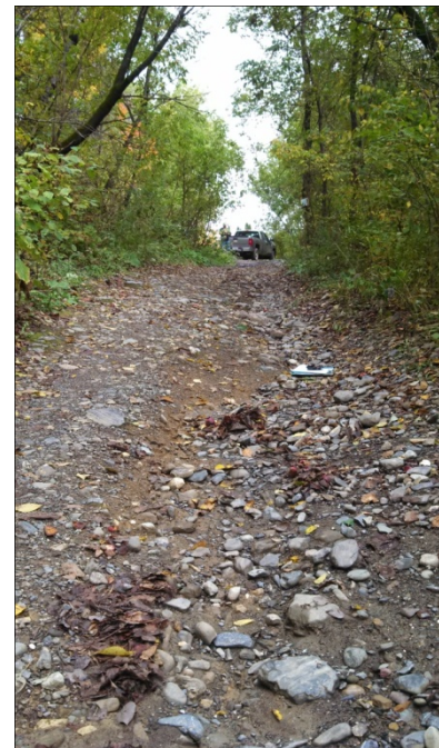
Gully erosion on an ATV trail with a 10% slope.
