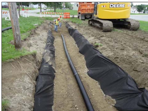
Downeast School biocell during construction.
