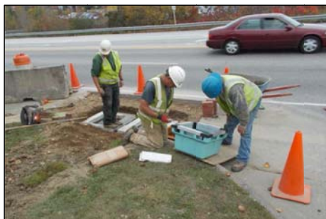
Crew installing a filter-equipped catch basin at the entrance to Swett's along Hogan Road.
