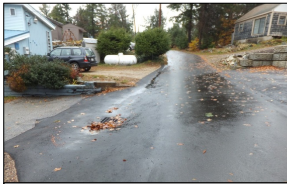
Langley Shores Road – 150 feet of steep gravel road was paved, and a catch basin was installed at the base to infiltrate runoff and capture sediment before it washes into the lake.
