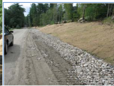
After – bank removed, slope stabilized, ditch installed
