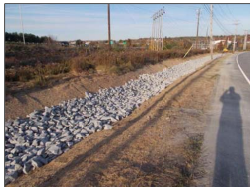
400 feet of linear ditch stabilized with filter fabric and riprap along Sylvan Road.
