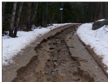
Erosion found during Toddy Pond watershed survey.
