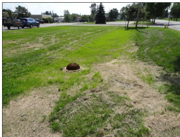
Downeast School biocell after construction.
