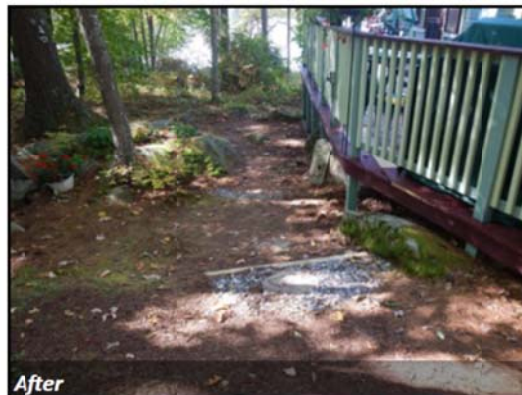
Erosion along this residential walkway was addressed using lumber and crushed stone to create steps or tiers, and bare soil was covered with three to four inches of erosion control mulch.
