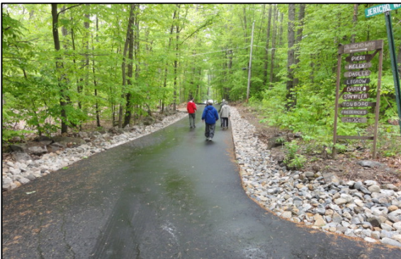
Abbott and Jericho Roads – 400’ of eroding gravel road was crowned and paved, and water redirected into ditches. The grant provided $3,500 and the road association provided almost $2,000 in match.
