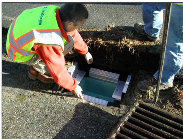
One of 12 filtration BMP catch basin inserts installed on Highland Avenue to trap phosphorus & other pollutants.
