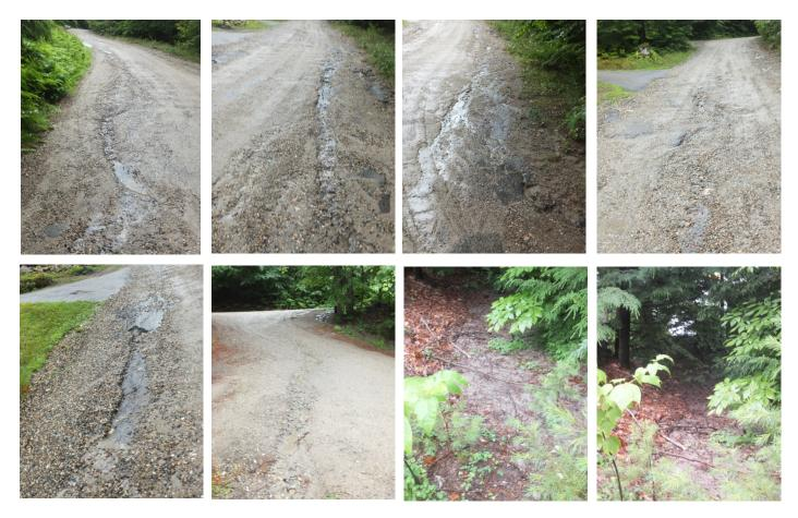
2. Intersection of Foley Way to 840 Lakeside Drive; <u>Private Road, Great East Lake.</u> Road site has severe road shoulder erosion, undersized ditch with severe erosion depositing runoff across private properties into Great East Lake. Recommendations include ditching and resurfacing approximately 700' of road and crown to divert runoff into ditches. Total Construction Cost: \$5,000 (\$3,000 grant, \$2,000 match)
