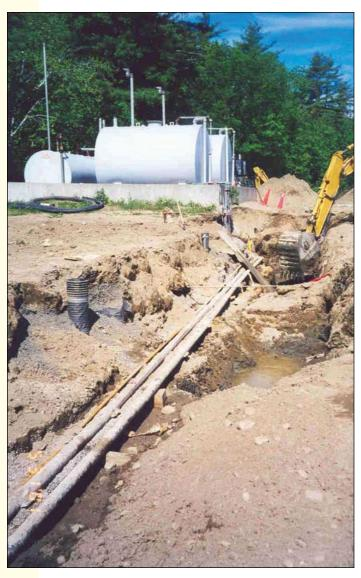
Underground piping associated with ASTs is a frequent source of leaks.
