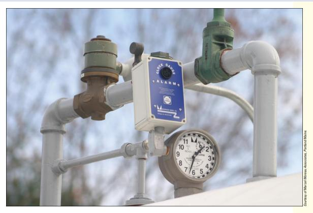
Overfill prevention for ASTs is very important. This tank is equipped with a gauge that can be easily read by the delivery person and a high level alarm.
