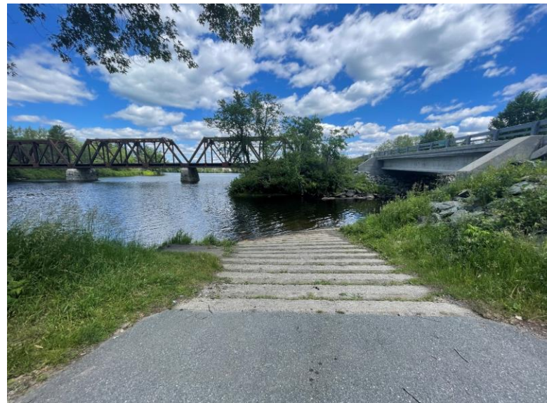
Site of DV-01 and EX-02 at confluence of the Johns and Connecticut Rivers (June 2021)
