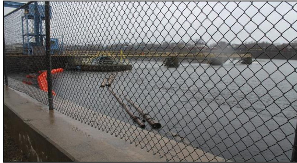
Existing boom positioned at dam intake on east side of river near location of EX-02.
