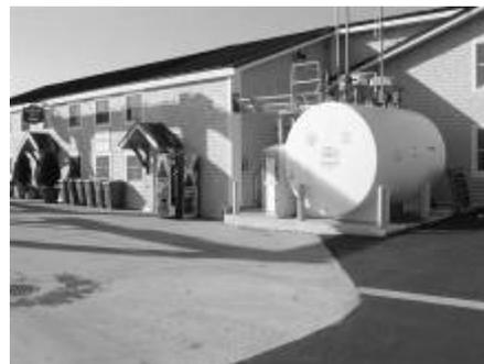
Double walled tank with protection
