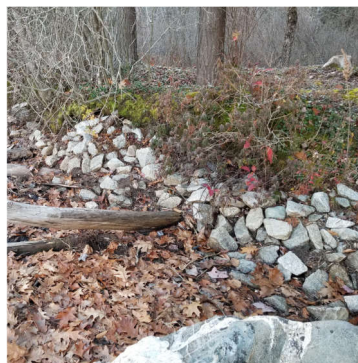
Toe riprap naturalizing as plants grow.
