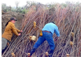
Brush bundles with posts.
