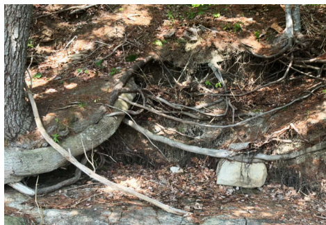
Evidence of toe erosion at a low-energy site, exposed during a period with a low water level.
