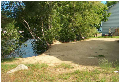
Evidence of sheet erosion (upper) and an eroding upland bank with lawn (lower).
