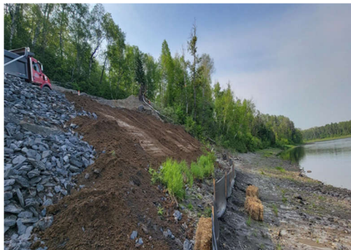
The riprap at this site is being infilled with soil. Then vegetation will be planted to increase stability.
