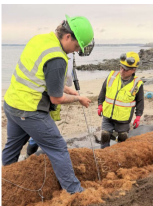
Anchoring a coir log. (Linkel)
