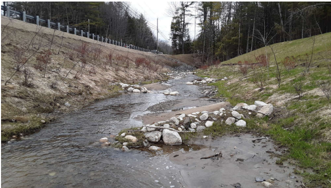
Groin in stream to slow flow in targeted areas.
