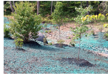
Hydraulically applied mulch.
