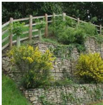
Vegetated gabion wall.
