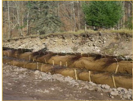
Upper: Fascine toe protection with live stakes. Lower: Encapsulated soil toe protection with brush layering.
