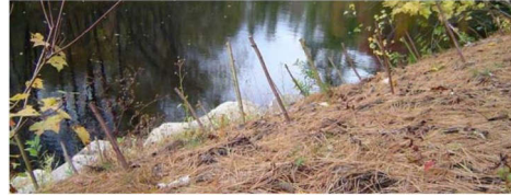
Live stakes installed on a shoreland slope.
