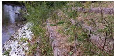
Encapsulated soil with live stakes soon after installation (upper) and after the live stakes began growing (lower).
