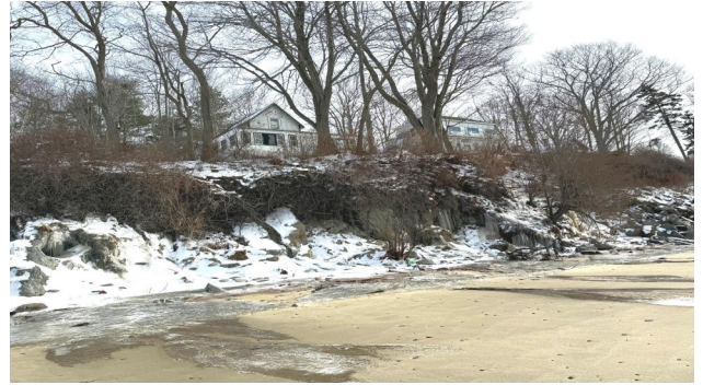
Groundwater instability and deflection from neighboring riprap Photo: P. Slovinsky, Maine Geological Survey
