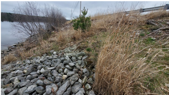
Edge of two stabilization projects. One with extended riprap and fabric (foreground) installed 1 year earlier than background that was graded and vegetated
