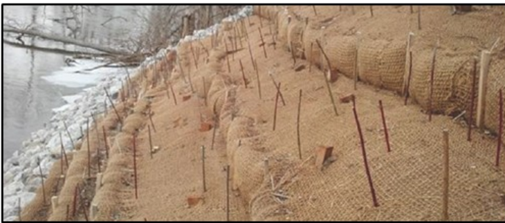
Slope stabilization using live stakes of dogwood & willow with coir blanket, slope interruption to control temporary erosion. Following construction and 1st growing season.
