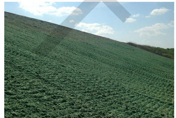
A roughened slope covered with hydroseed
