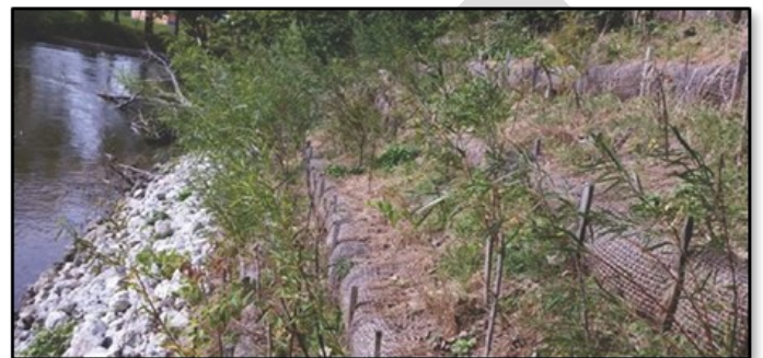
Slope stabilization using live stakes of dogwood & willow with coir blanket, slope interruption to control temporary erosion. Following construction and 1st growing season.
