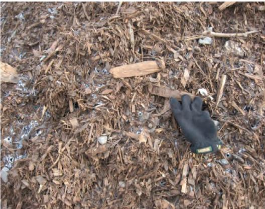
Erosion control mix consists primarily of organic material manufactured on or off the project site and may include: shredded bark, stump grindings, or partially composted wood products.
