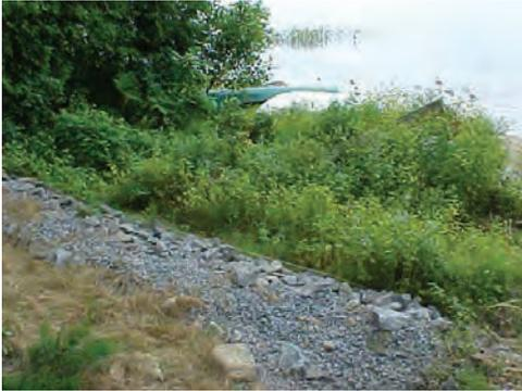
Level spreaders should be constructed on undisturbed soil. The buffer and area below the spreader should remain uncompacted from construction equipment.
