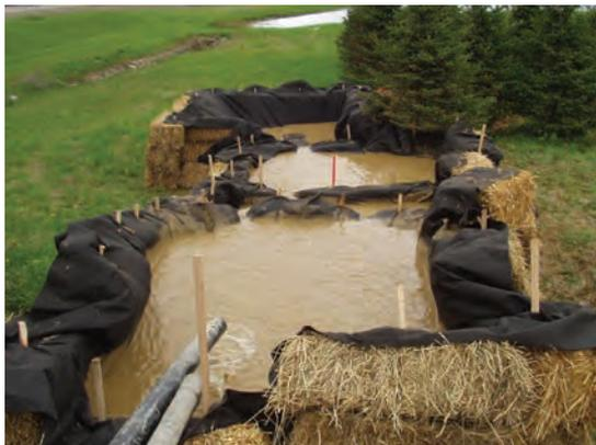
**NATURAL DEPRESSIONS** or excavated basins may be adapted to detain runoff. A low point in a natural depression could be blocked off by a temporary embankment (berm or sand bags) to increase its capacity. The embankment should be high enough to detain the expected volume of water, wide enough to resist collapse; and be appropriately stabilized.
