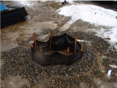
**SILT FENCE WITH GRAVEL** may be placed around the perimeter of a catchbasin and surrounded with gravel.
