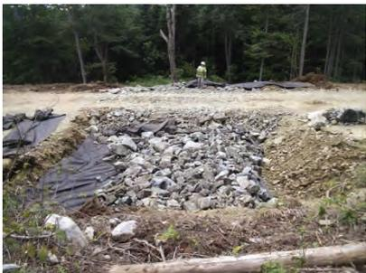
A rock sandwich can provide a permeable road base if built of coarse rocks and wrapped in geotextile fabric to let water drain downgradient.
