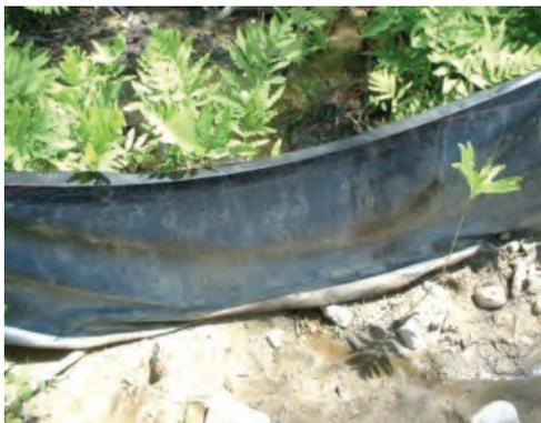
Silt fence can be difficult to install properly in shallow-to-ledge, stony, or forested soils as well as frozen ground. The added disturbance near a water resource is not recommended.
