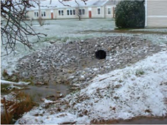
An apron protects and stabilizes the culvert outlet the full width of the bottom and one foot above the maximum outflow elevation.
