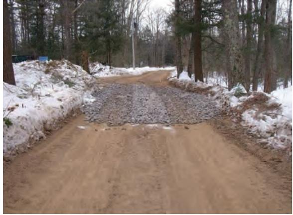
**TEMPORARY FORDS** consist of the reinforcement of the streambed for traffic while maintaining adequate fish passage but should not be used for streams with soft mucky bottom
