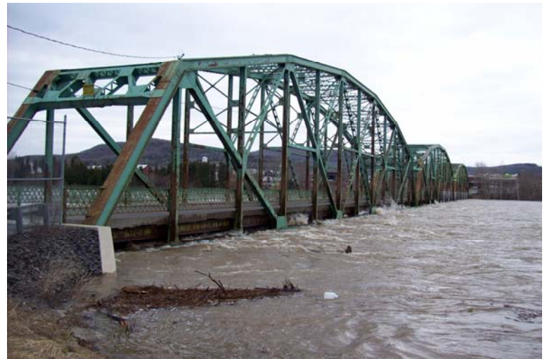
St. John River at Ft. Kent, Maine Flood 2008 (Photo credit: USGS)
