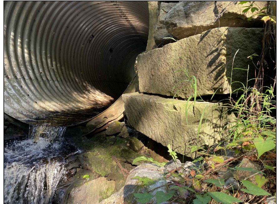
Inlet showing base of headwall shifted forward.
