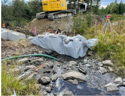
Cofferdam and pump intake during construction
