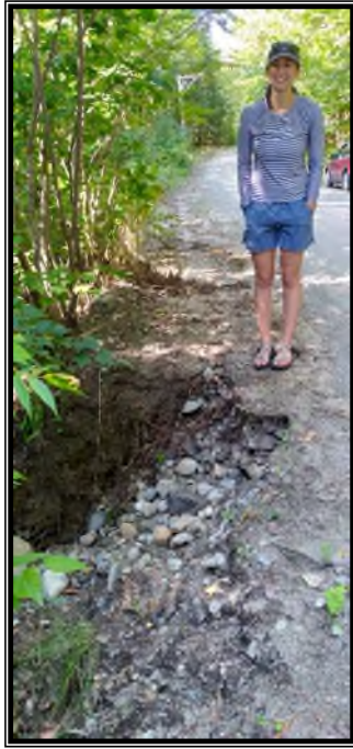
Picture #9: View of eroded road embankment from September 13, 2021
