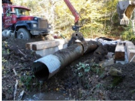
Removal of existing culvert
