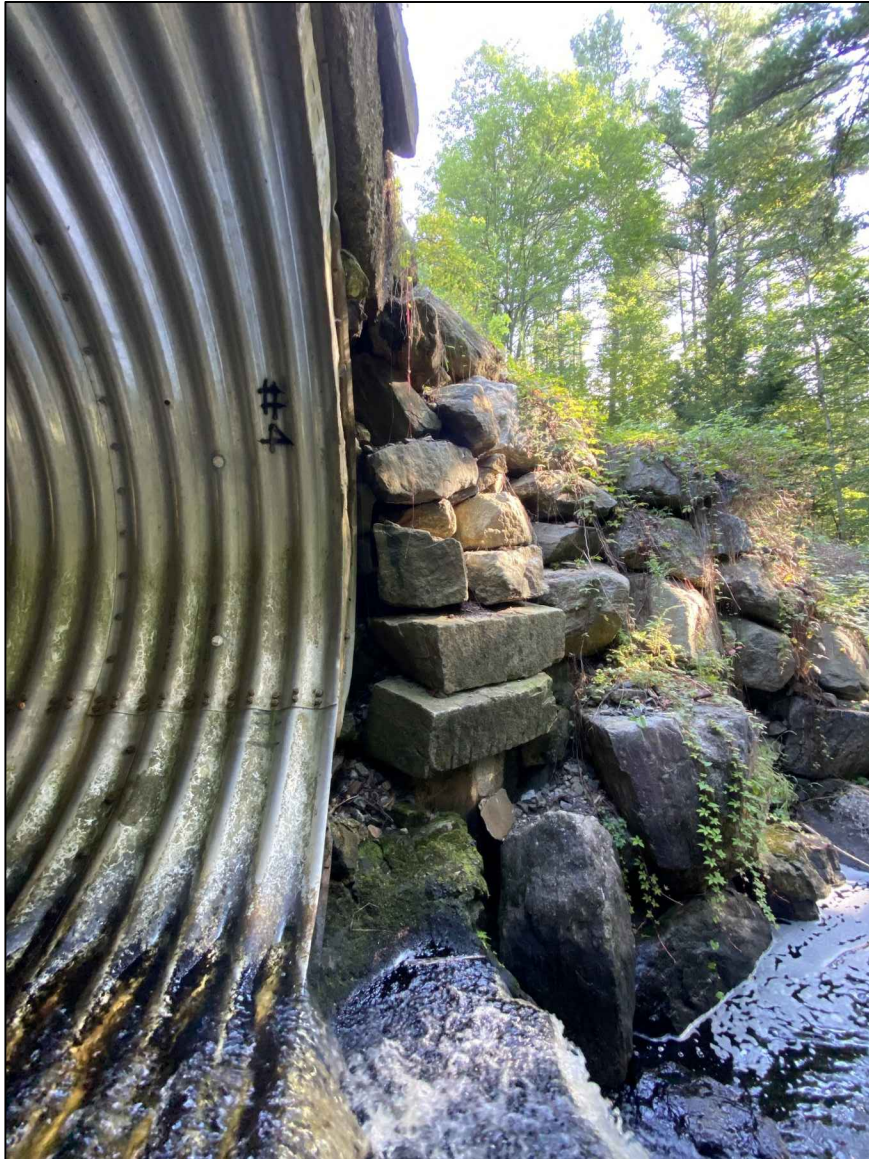
Inlet showing base of headwall shifted.
