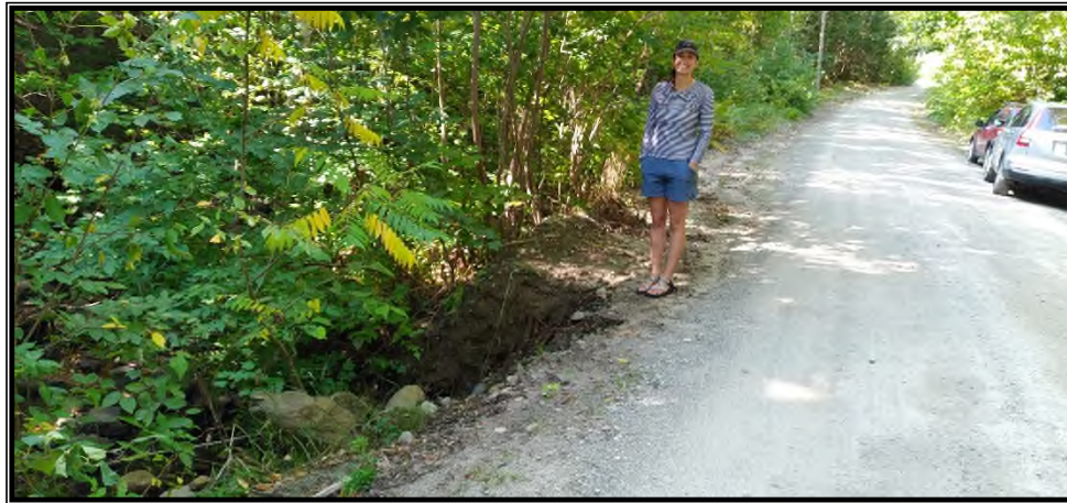
Picture #10: View of eroded road embankment from September 13, 2021
