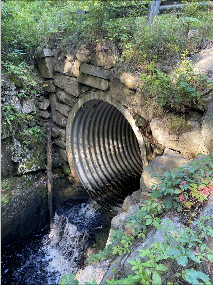
Outlet showing failing headwall.
