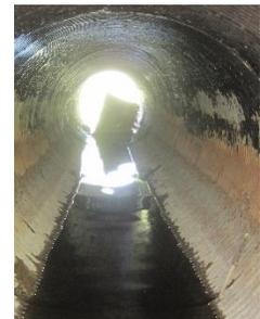
Figure 3 Bent up end
