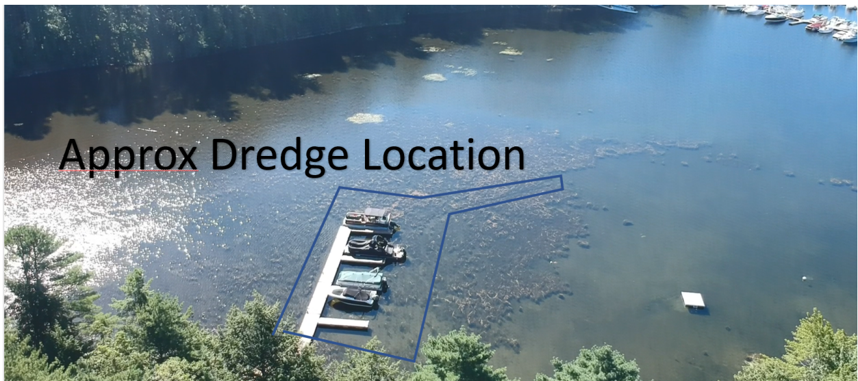
Figure 13. - Aerial View of KCOA dock
