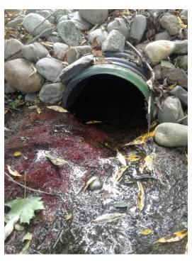
Fig. 2. This outfall is partially submerged and a clean catch of its discharge is not possible.
