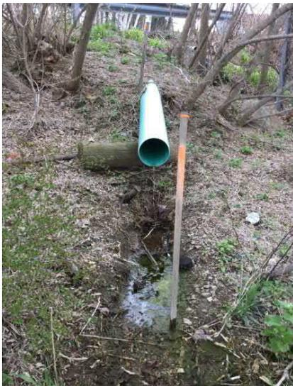
*This outfall, though in poor condition because it is cantilevered, provides a good opportunity for a clean catch of its discharge.*
