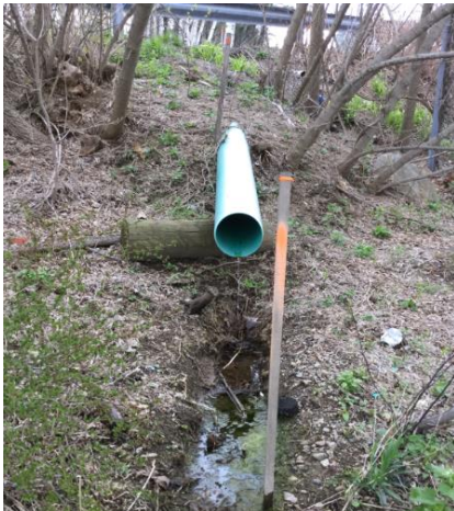
This outfall, though in poor condition because it is cantilevered, provides a good opportunity for a clean catch of its discharge.
