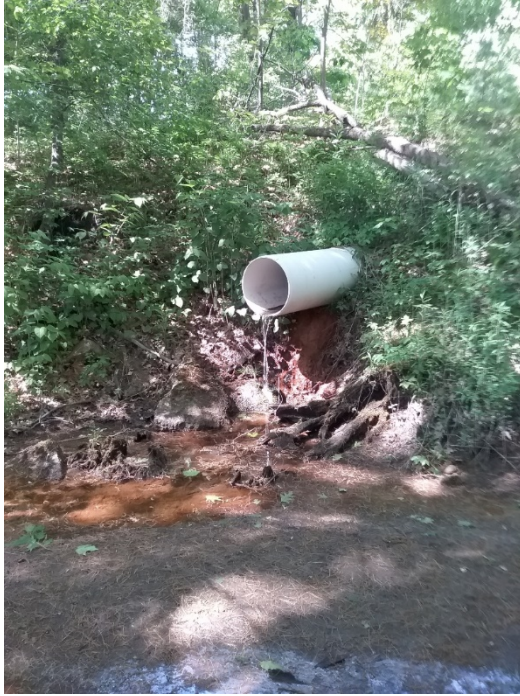
Fig. 1. This outfall provides a good opportunity for a clean catch of its discharge.
