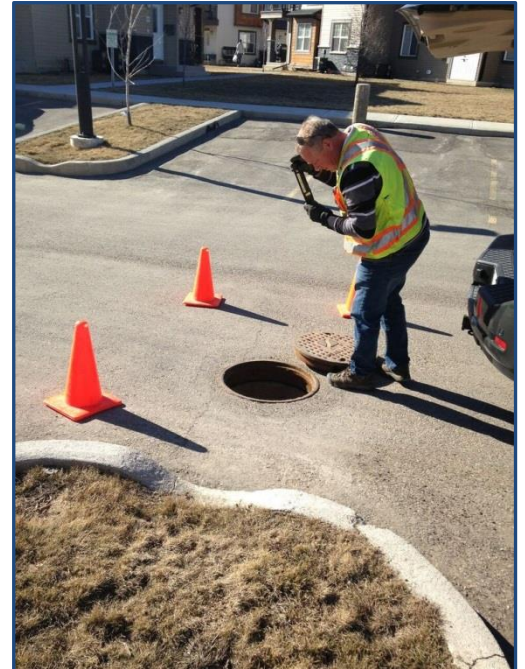
Source: Pro-Hawk Inspections
