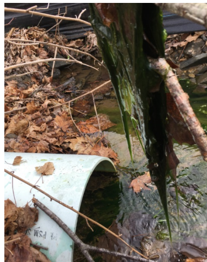
This outfall is partially submerged and a clean catch of its discharge is not possible. If tidal influences are strong, wait until low tide to sample. Additional options include: sampling upstream structures or using sand bags around the outfall to prevent contamination from backflow.
