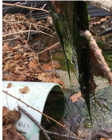
This outfall is partially submerged, and a clean catch of its discharge is not possible. If tidal influences are strong, wait until low tide to sample. Additional options include: sampling upstream structures or using sand bags around the outfall to prevent contamination from backflow.
