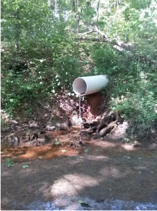
Fig. 1. This outfall provides a good opportunity for a clean catch of its discharge.
