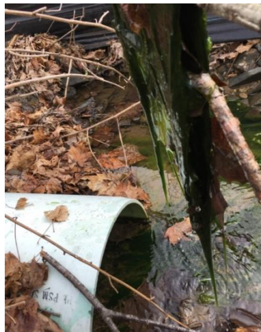
This outfall is partially submerged, and a sample of its discharge is not possible. If tidal influences are strong, wait until low tide to sample. Additional options include sampling upstream structures or using sand bags around the outfall to prevent contamination from backflow.
