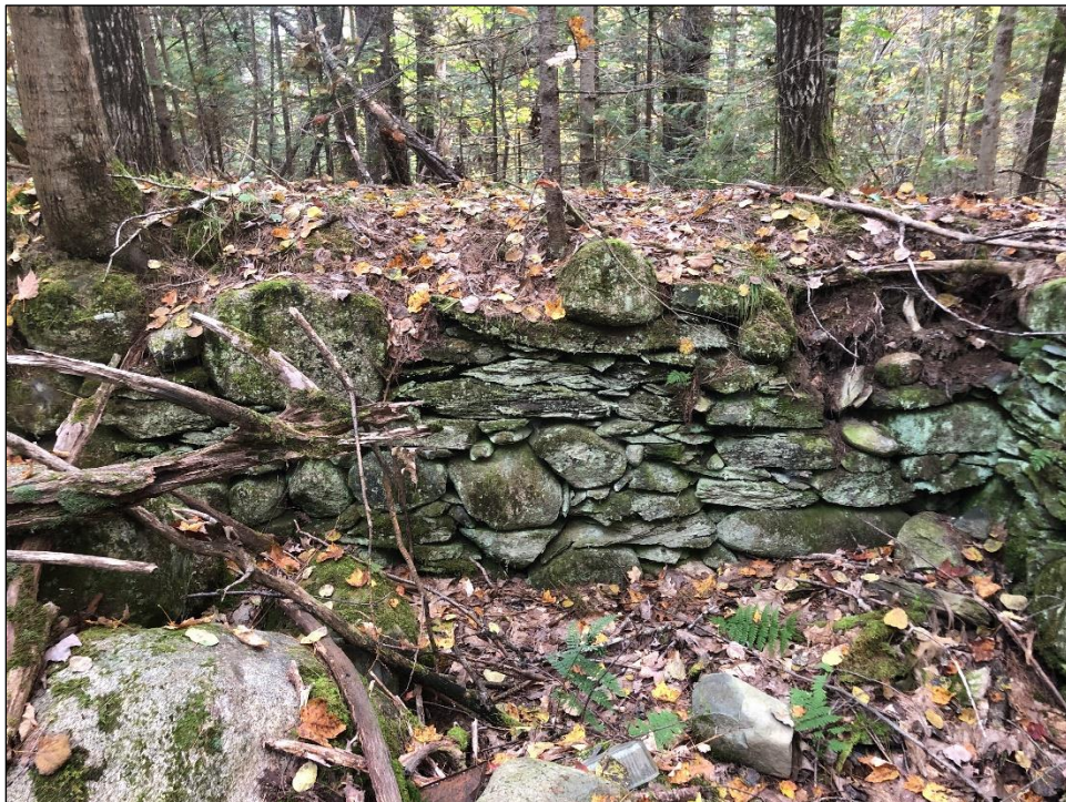
Figure 5-49. North wall of cellar hole at Site ME 038-003, looking north.
