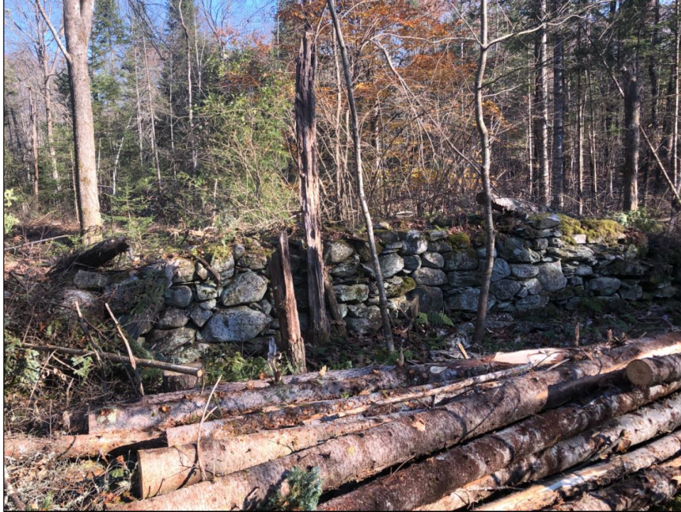
Figure 5-58. Intact southern wall of structure at Site ME 441-005, facing northeast.
