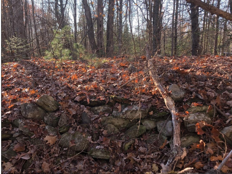
Figure 5-9. Northeast portion of Site ME 097-007 structure east wall, facing west.
