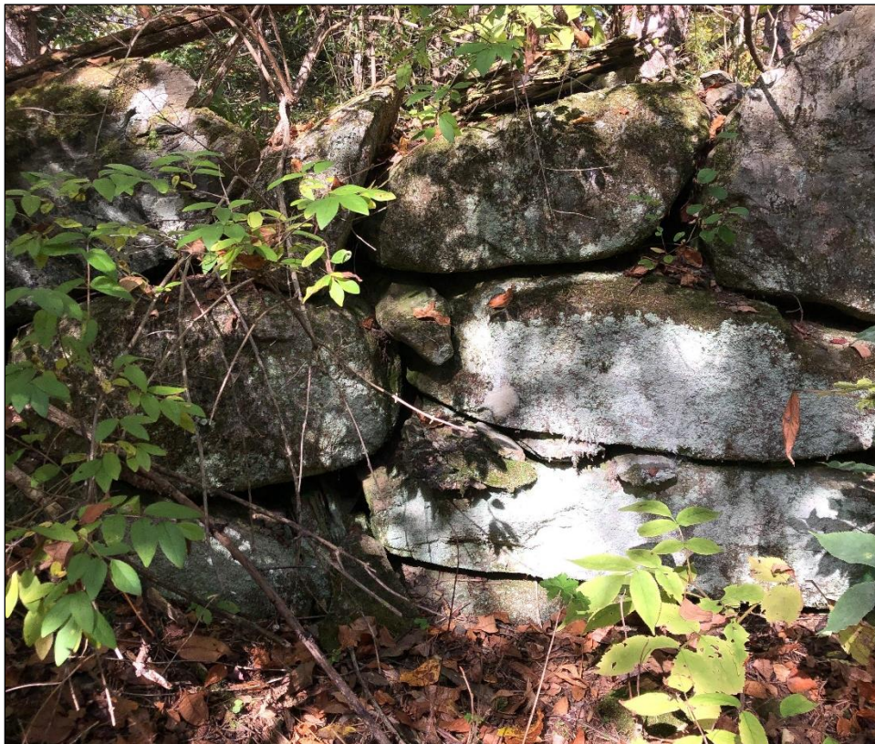
Figure 5-25. North wall of the Site ME 097-004 foundation, facing north.
