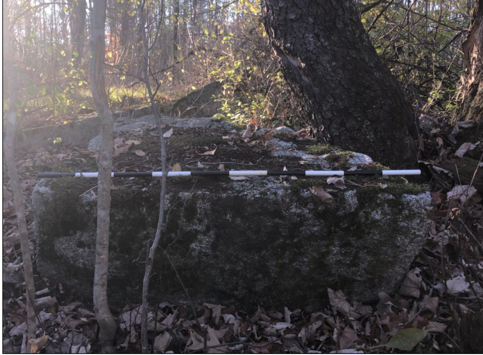
Figure 5-15. Southeast corner of footer at Site ME 097-008, facing west.
