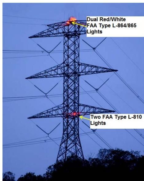
Figure 16. The FAA Type L-864/L-865 Obstruction Lights Controlled by the HARRIER ADLS [3]
