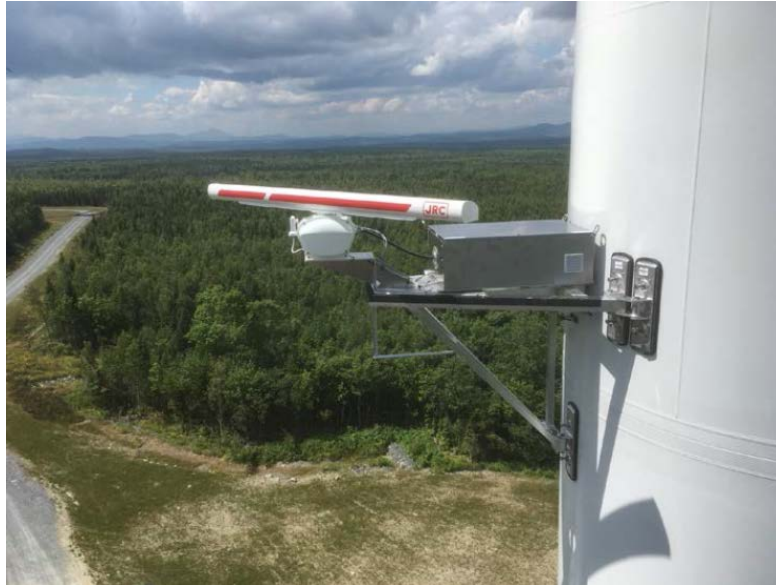
Figure 15. Example of Radar Installed at Hancock Wind Project [7]
