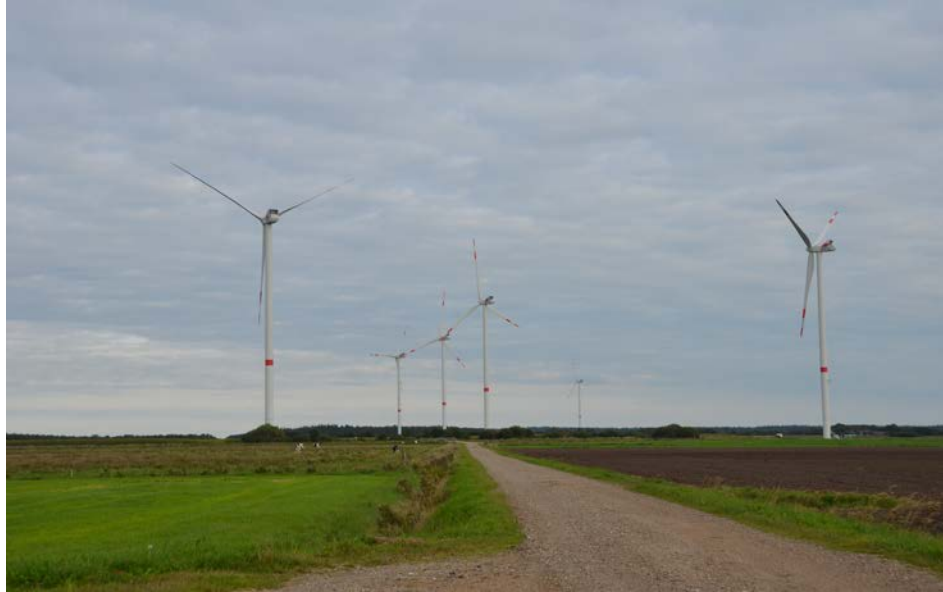
Figure 6. Wind Turbines at the Braderup Wind Park
