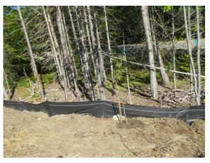
control mix berms or placement of six inches of suitable non-organic material along fabric flap on upslope side of fence, in lieu of burying fabric in trench.
