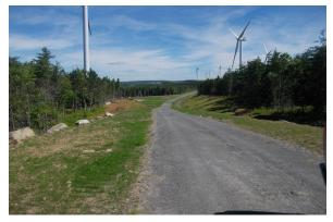
section or swale on the downhill side of the permanent road, within the original 24, 34, or 40-foot-wide area. In other words, the permanent road section includes a 2-foot wide vegetated shoulder on the uphill side, 12-foot wide gravel maintenance road, and 20 to 28-foot wide vegetated level buffer edge and treatment swale on the downhill side.
