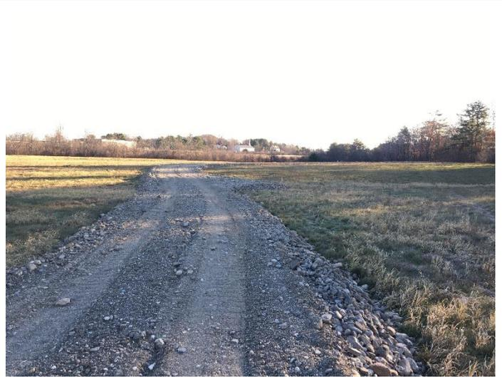
Photo 20 (11/12/18): View, looking east, of the gravel road constructed in the Site hayfield for drill rig access.
