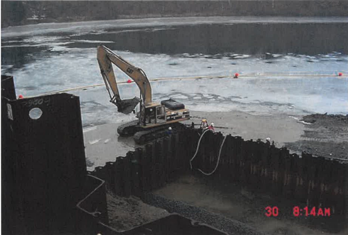
Example of a shoreline coffer cell and excavator on the mudflats.
