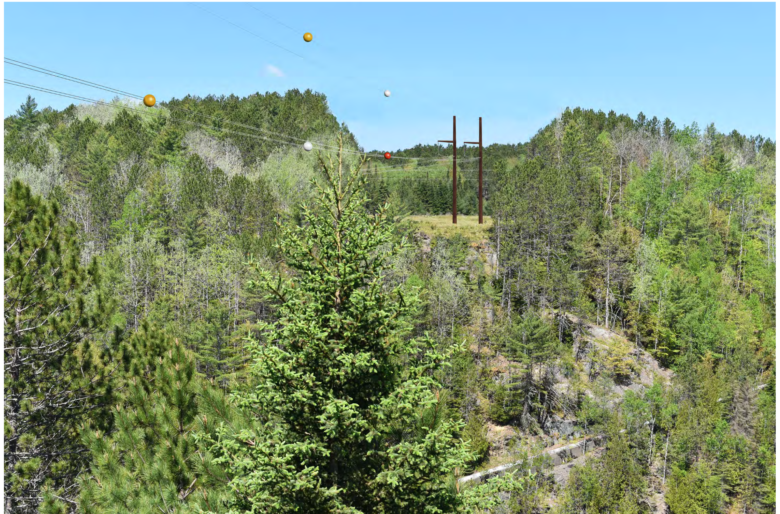
Proposed Conditions: Normal view looking northwest from the top of the Kennebec River access steps adjacent to Harris Dam. Due to the steep topography and required clearing, one 85' HVDC structure would be entirely visible on the north side of the river, 880 feet from this viewpoint. The proposed clearing would reveal an additional portion of the existing Jackman Tie Line transmission corridor behind the proposed structure.
