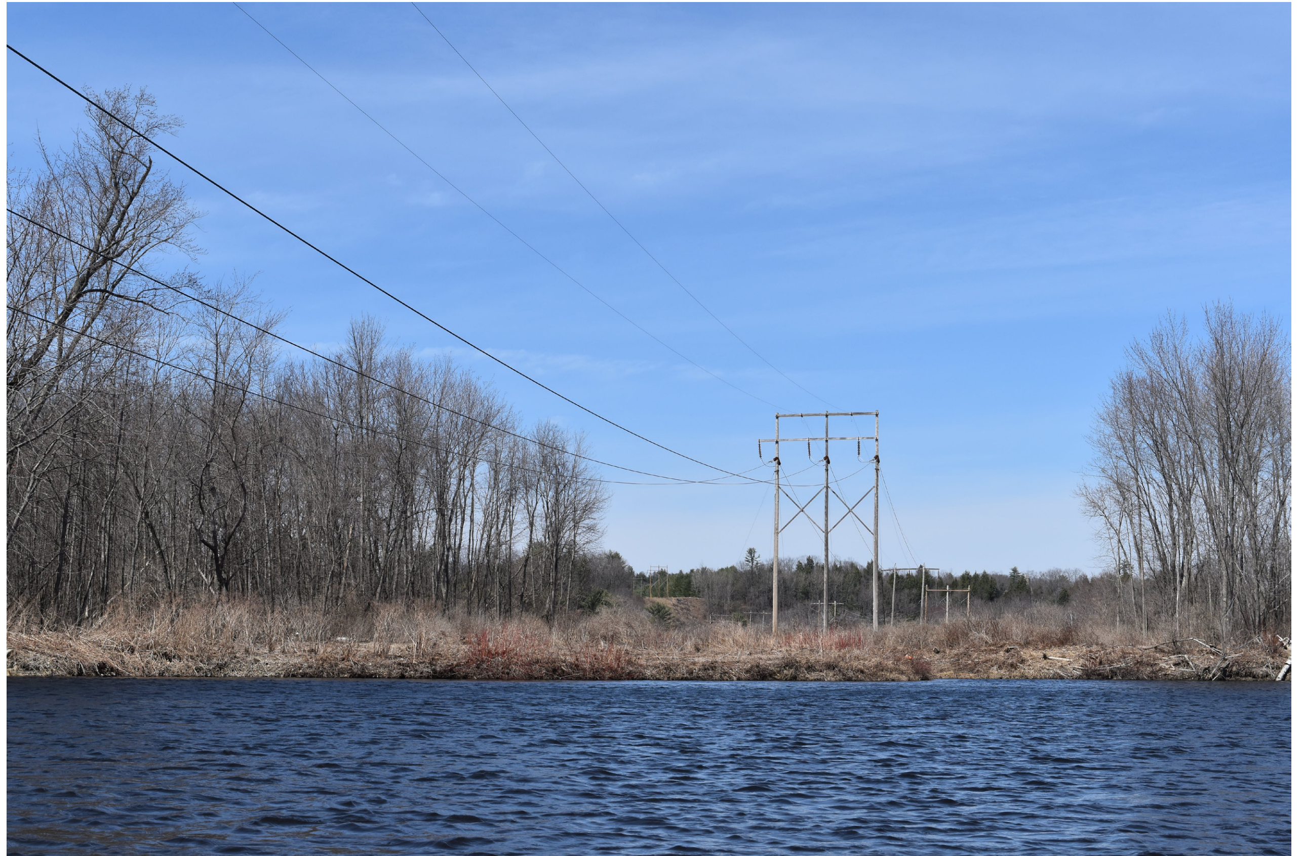
Existing Conditions: Normal view looking north from the Carrabassett River in Anson toward the existing 115 kV transmission line.
