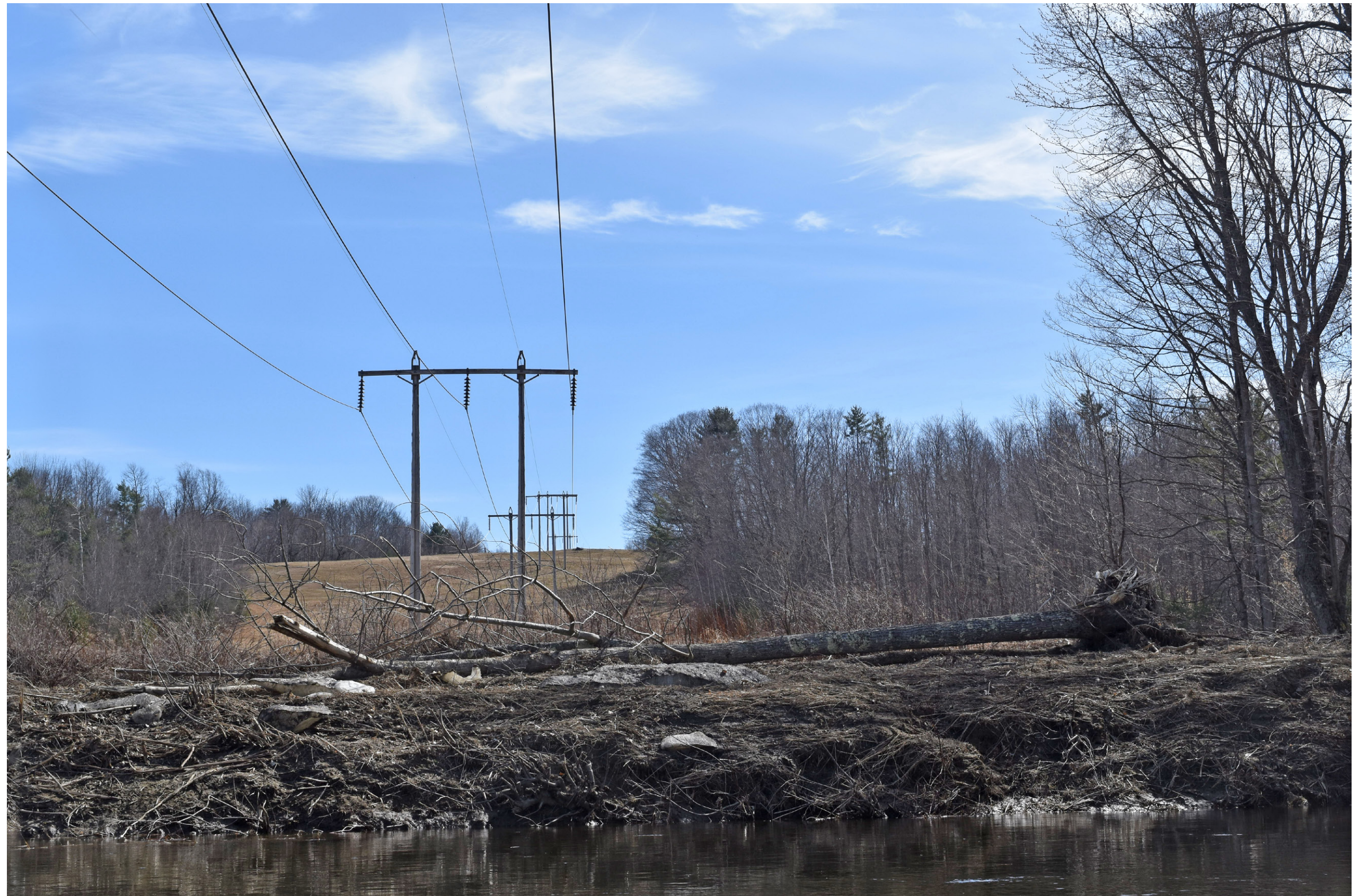
Existing Conditions: Normal view looking south from the Sandy River in Farmington toward the existing 115 kV transmission line.
