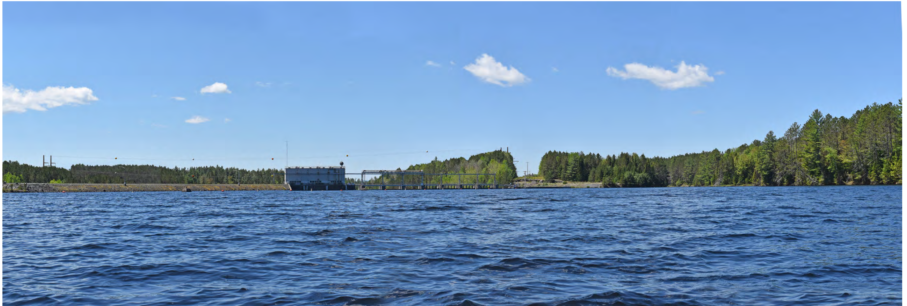
Proposed Conditions: Panoramic view looking south to west from Indian Pond Impoundment toward the Harris Dam and existing Jackman Tie Line transmission corridor. Portions of five proposed HVDC structures would be visible at distances of approximately 1,810 to 3,100 feet from this location.
