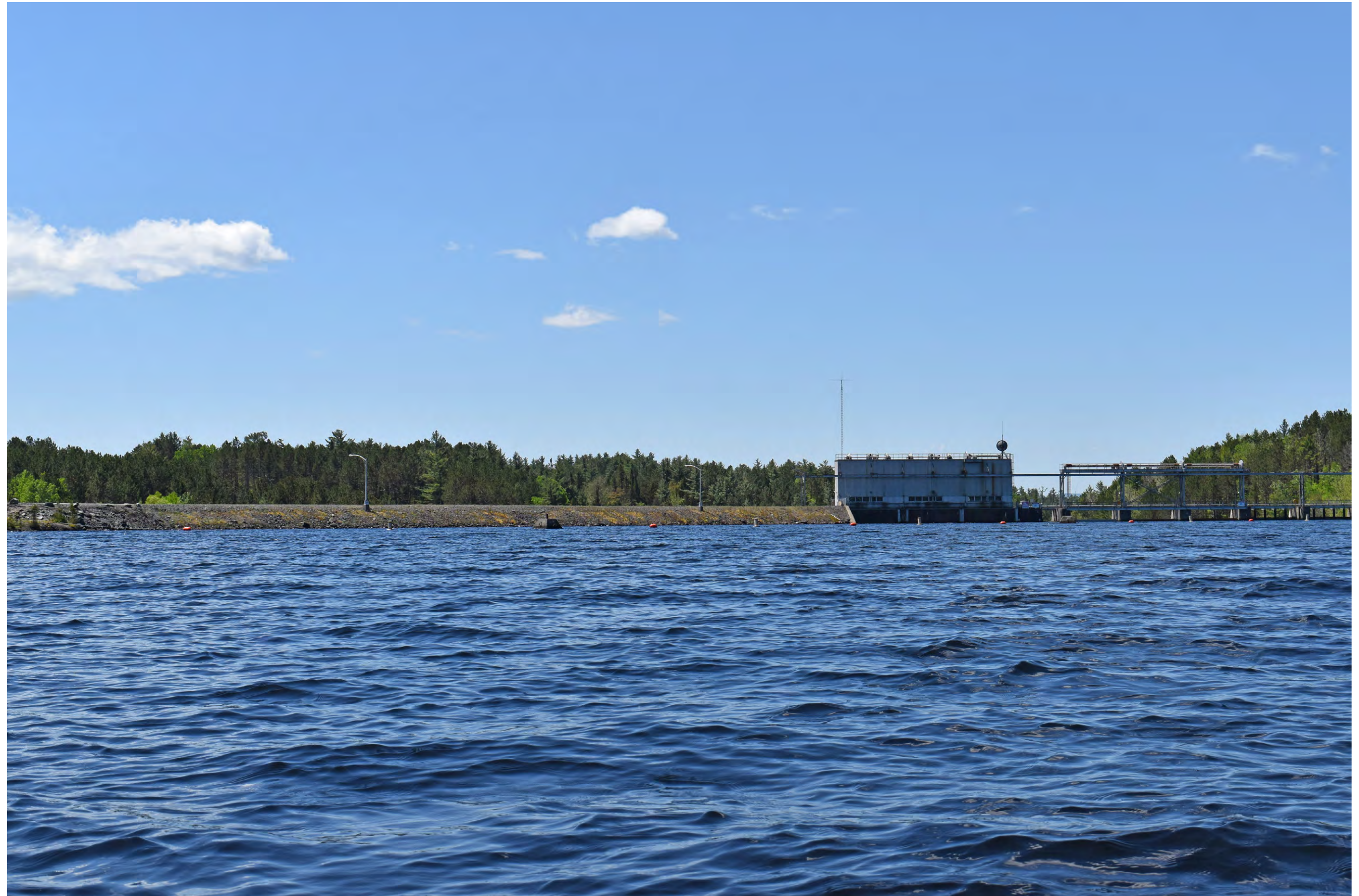
Existing Conditions: Normal view looking southwest from Indian Pond Impoundment toward the Harris Dam.
