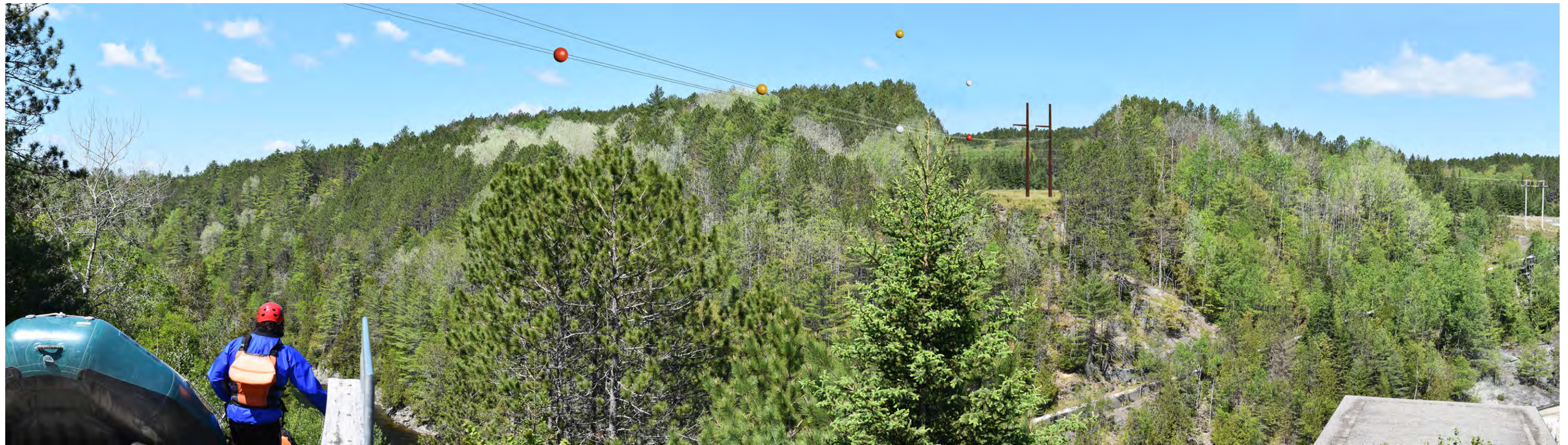
Proposed Conditions: Panoramic view looking west to northwest from the top of the Kennebec River access stair adjacent to the Harris Dam. The roof of the powerhouse, a concrete sluiceway, and a portion of the Jackman Tie Line are visible in this image. One proposed 85' HVDC structure would be visible across the river approximately 880 feet from this location. The conductors would be approximately 180' above the water level. Shield wires and conductors with marker balls would pass directly over the access stairs. Approximately 325' of vegetation below the visible structure within the 150' wide corridor would be removed to maintain clearance for the conductor safety zone. Approximately 105' of vegetation would remain adjacent to the river on the northwest side, and 150' on the southeast side.
