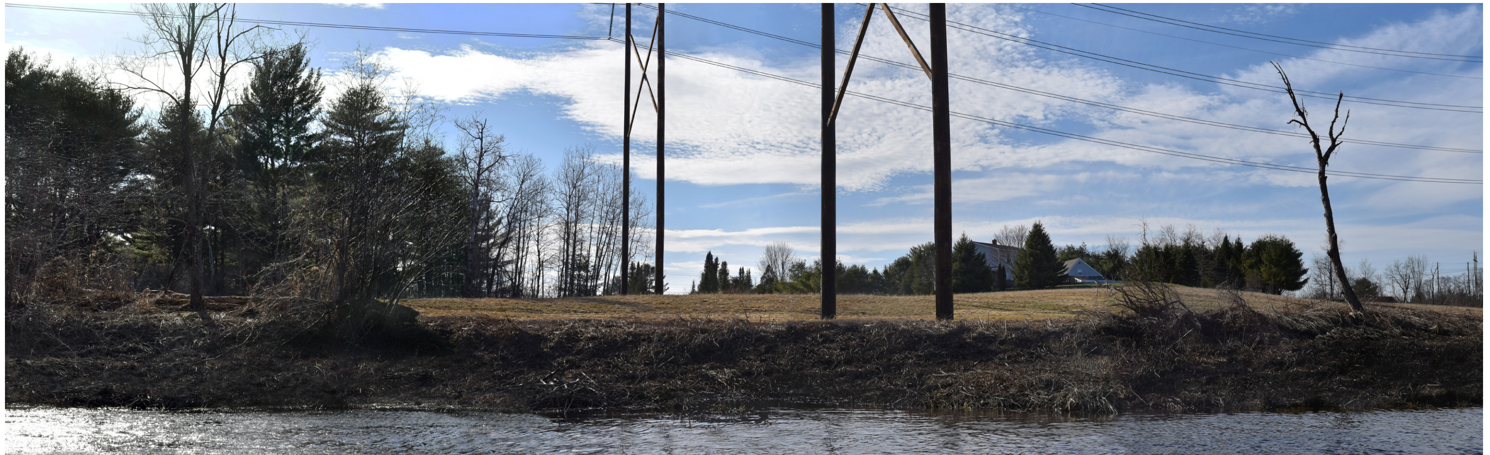
Proposed Conditions: Panoramic view looking west to north from the West Branch Sheepscot River in Windsor toward the proposed co-located 345 kV transmission line (see continuation of this view to the north, Photosimulation 36). The existing 345 kV transmission line will be relocated 40' to the west to accommodate the proposed 345 kV transmission line. One proposed 345 kV structure and conductors will be visible approximately 112 feet from this viewpoint. No additional vegetation will be removed in this area directly adjacent to the river.
