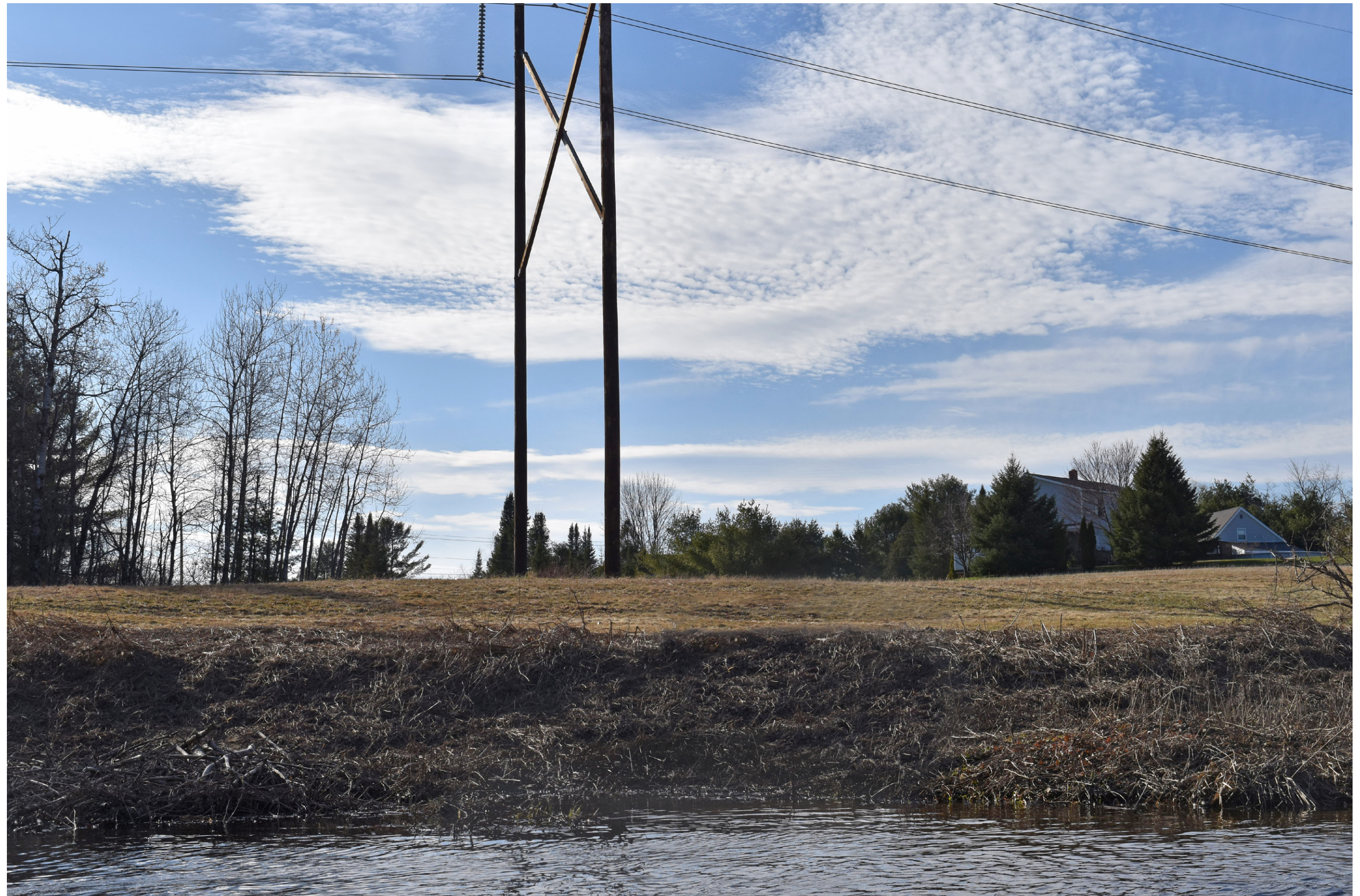
Existing Conditions: Normal view looking west from the West Branch Sheepscot River in Windsor toward the existing 345 kV transmission line.
