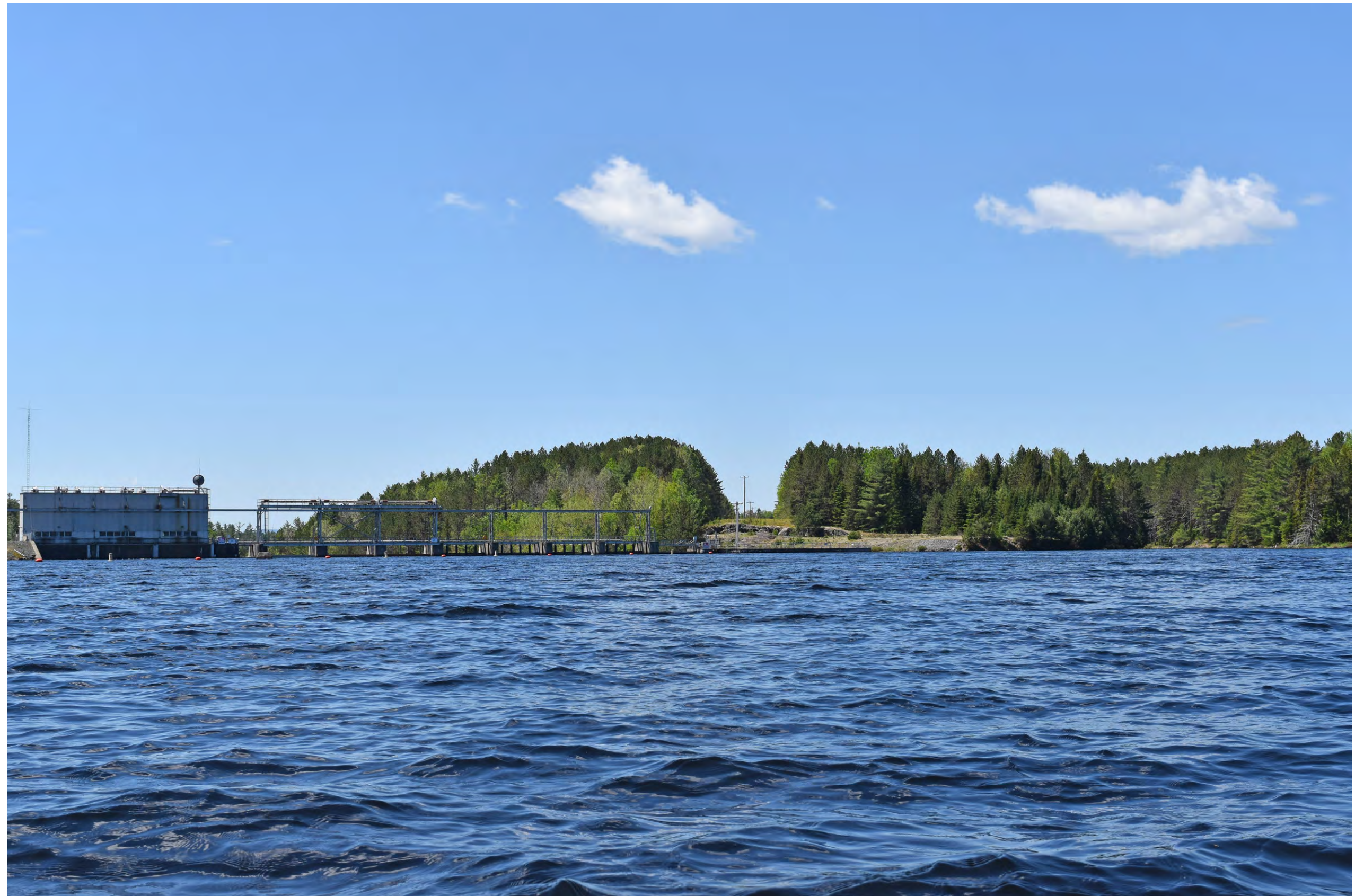
Existing Conditions: Normal view looking west from Indian Pond Impoundment toward the Harris Dam and the existing Jackman Tie Line transmission corridor.
