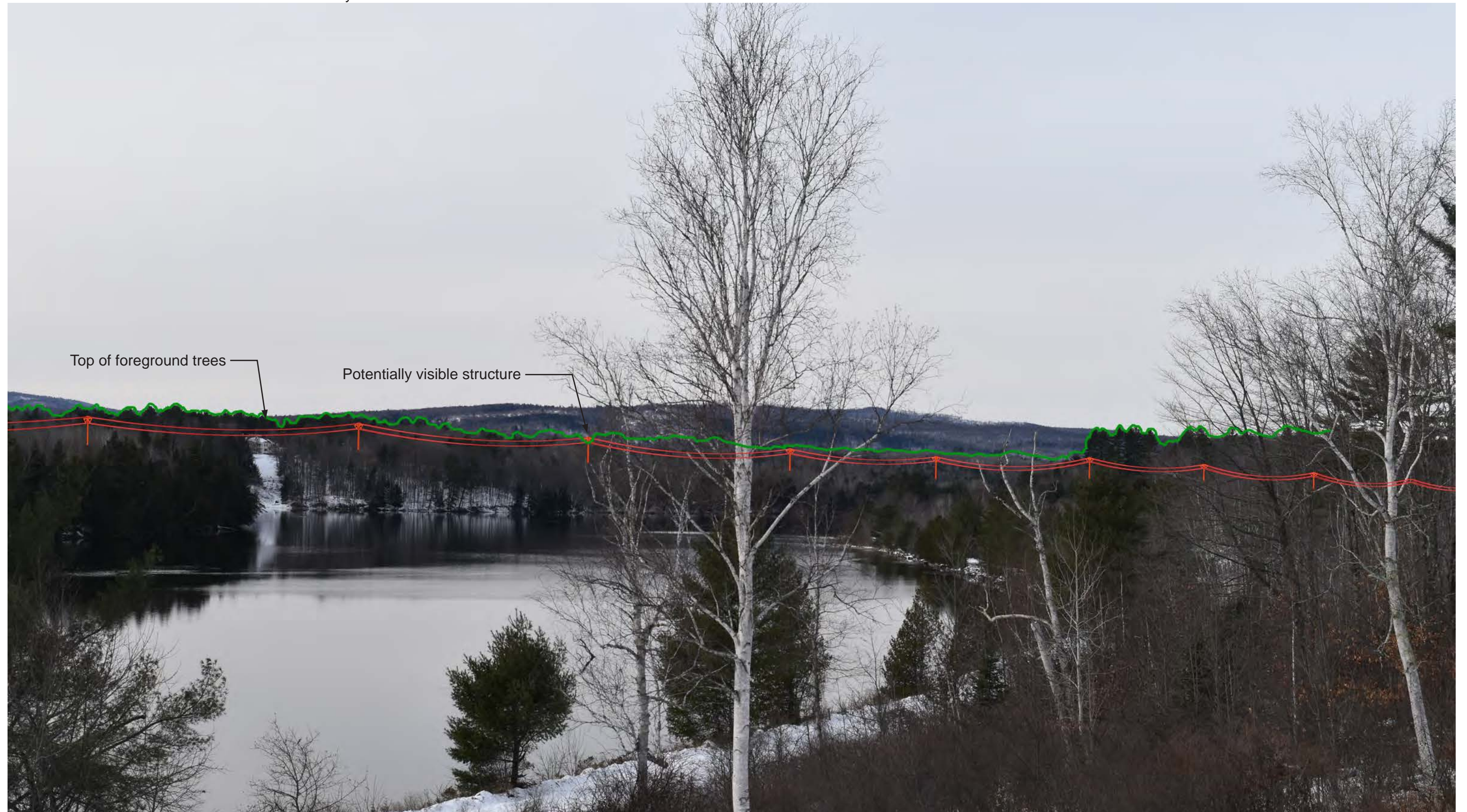
Viewpoint 7 (model overlay) - View looking northwest from the Route 201 Overlook in Solon toward the Project. The top of one structure may be visible from this viewpoint. Red lines represent conductors that are located behind the existing vegetation, except in one location as noted.
