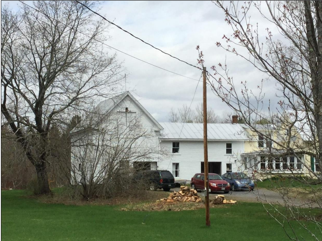
Figure 2. Connected barn (ID-1126) at 23 Horseback Road
