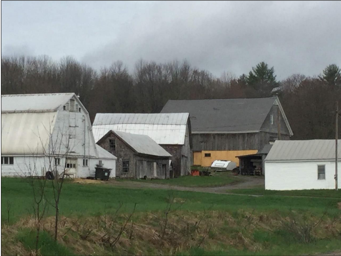
Figure 4. Outbuildings at E. Gray Farm, 1294 Anson Road, Starks
