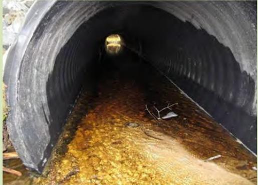
***A culvert installed to stream smart principles that is accumulating substrate***
