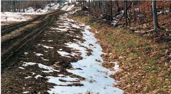
*Revegetated road ditches carry water without eroding.*
