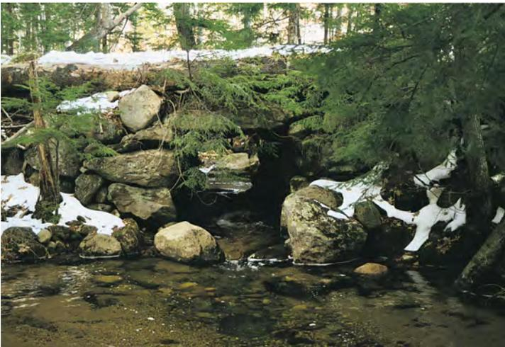
*An old stone culvert still functioning.*
