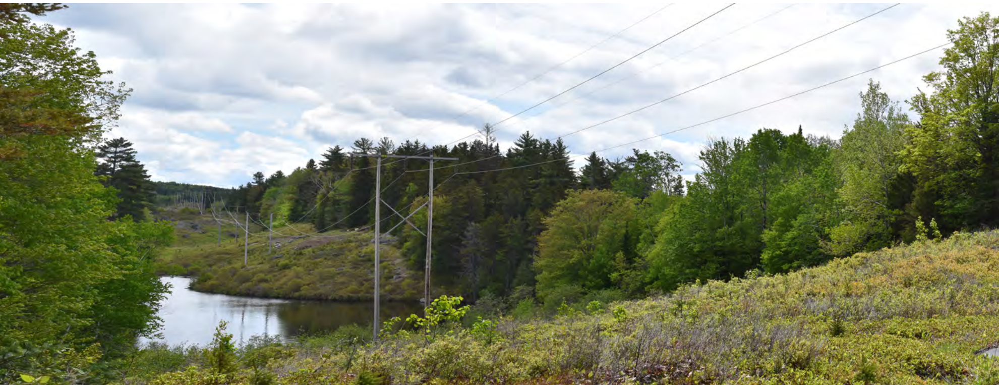
VP5.B: Panoramic view looking southeast towards Joe’s Hole (Moxie Pond) at the intersection of the Appalachian Trail and the existing transmission line corridor. The existing 150’ wide transmission line clearing will be widened by 75’ on the western side (to right of clearing in image above) to accommodate the new HVDC transmission line corridor. Portions of six self weathering steel HVDC structures will be visible from this viewpoint. See Photosimulation B.
