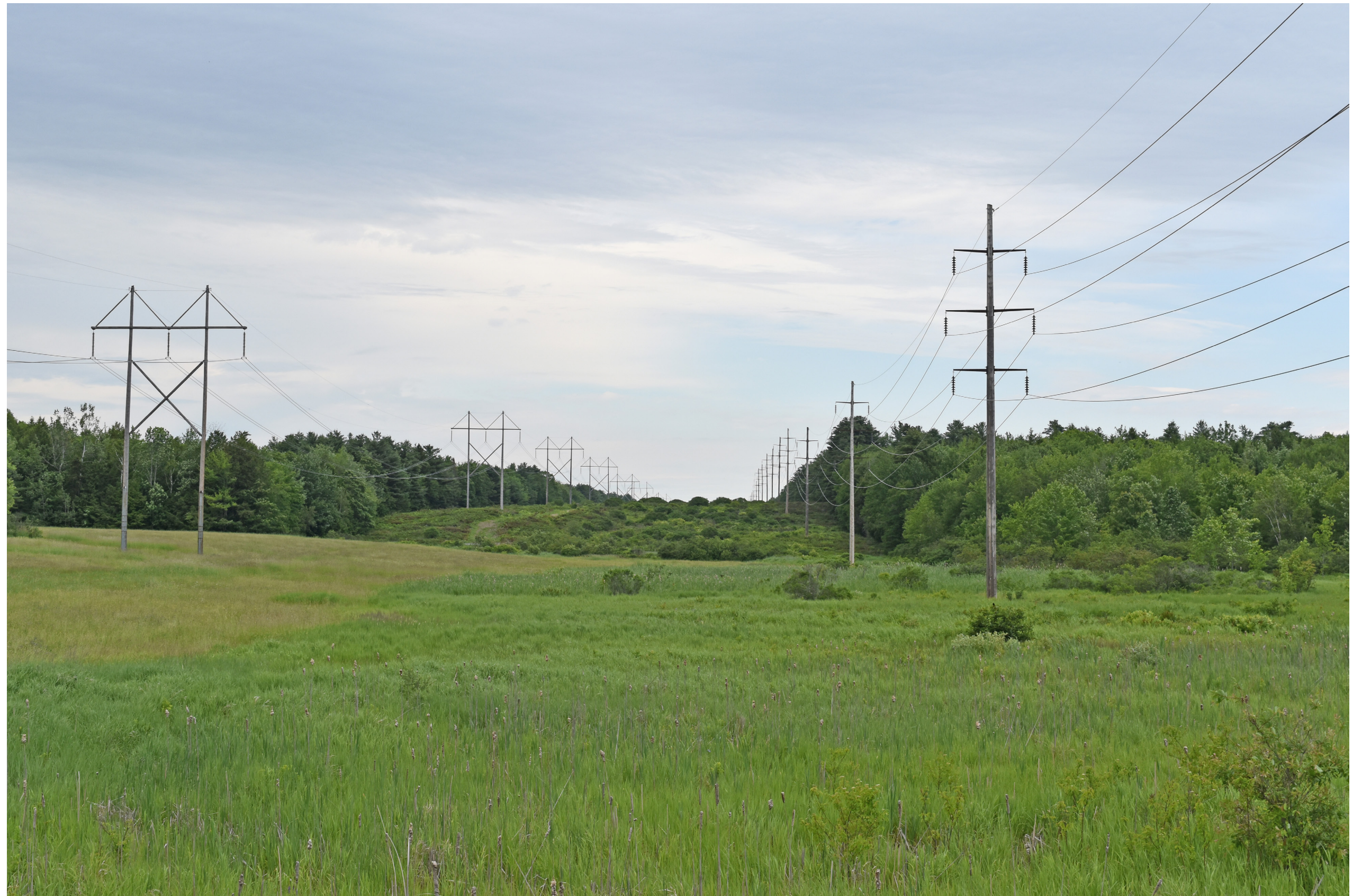
Existing Conditions: Normal view looking from north to northeast from Route 27.
