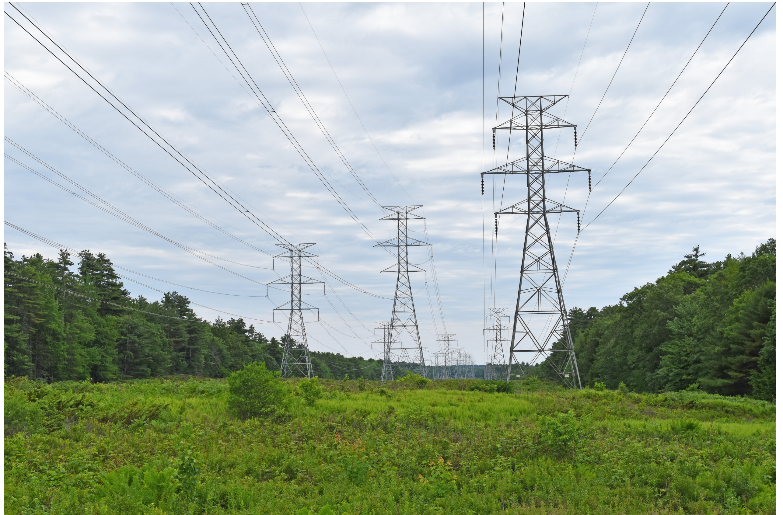
Existing Conditions: Normal view looking south from Route One in Wiscasset towards the existing 115 kV and 345 kV transmission lines.
