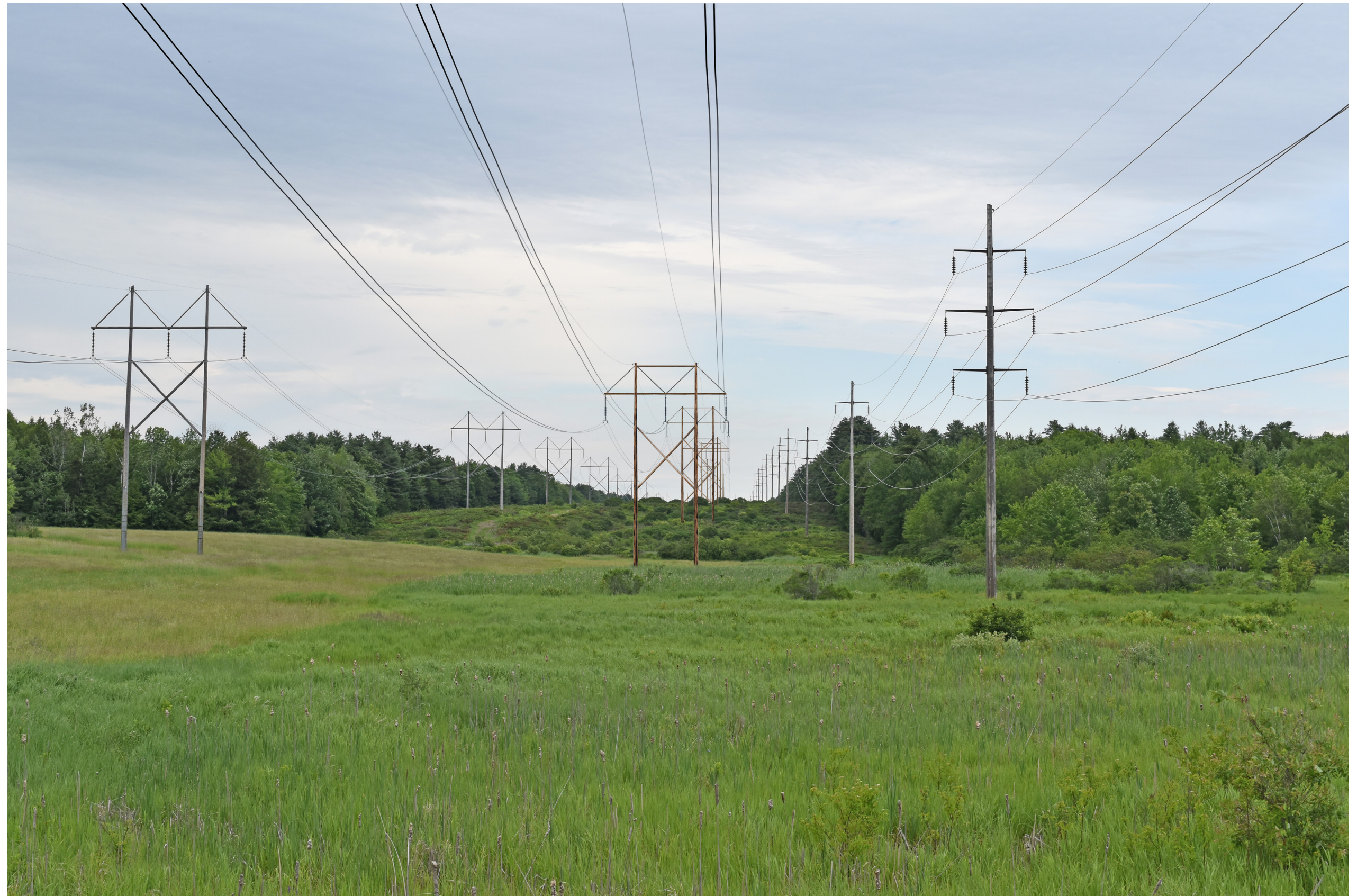
Proposed Conditions: Normal view looking from north to northeast from Route 27 toward the proposed co-located 345 kV transmission line. The proposed 345 kV transmission line will be located in between the existing 115 kV and 345 kV transmission lines. Seven structures and conductors will be visible from this viewpoint.
