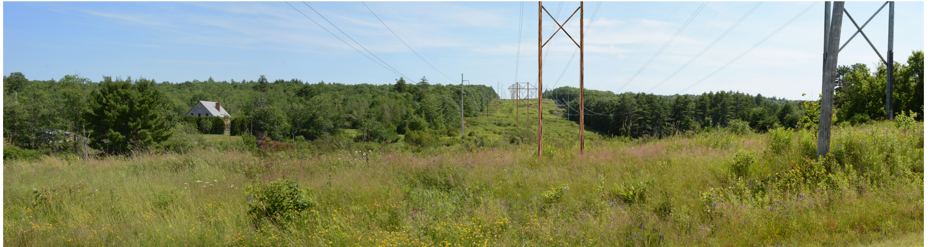
Proposed Conditions: Panoramic view looking from southeast to southwest from Route 194 toward the proposed co-located 345 kV transmission line. The proposed 345 kV transmission line will be located in between the existing 115 kV and 345 kV transmission lines. Seven structures and conductors will be visible from this viewpoint. See Appendix B: Study Area Photographs for additional images.
