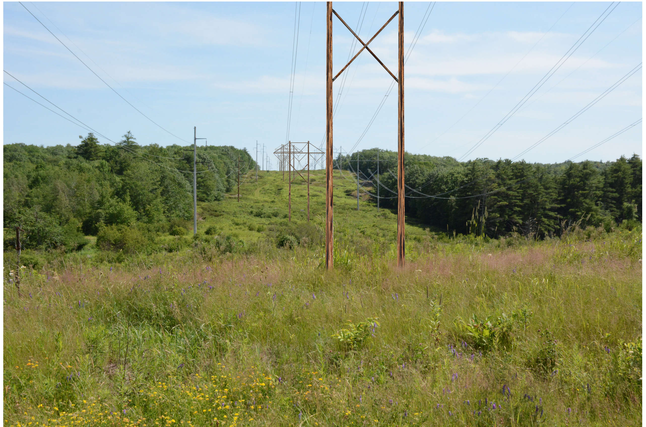
Proposed Conditions: Normal view looking from southeast to southwest from Route 194 toward the proposed co-located 345 kV transmission line. Seven structures and conductors will be visible from this viewpoint. The proposed 345 kV transmission line will be located in between the existing 115 kV and 345 kV transmission lines.
