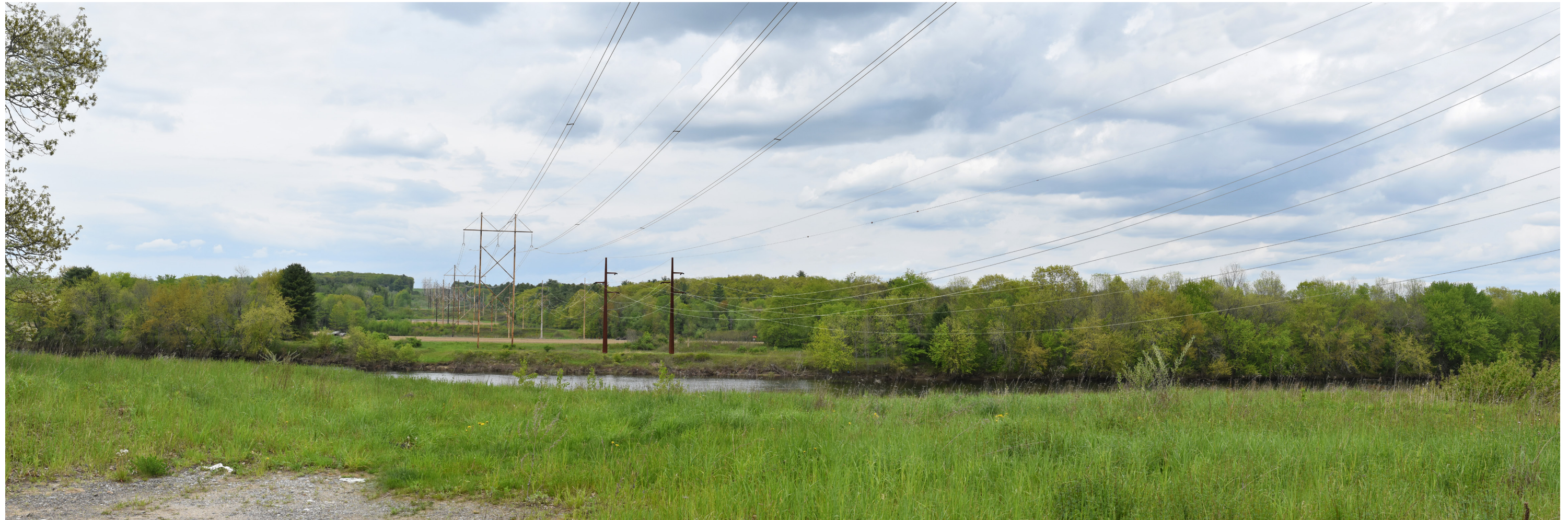
Proposed Conditions: Panoramic view looking from north to northeast from Riverside Drive / Route 136 in Auburn over the Androscoggin River toward the proposed Sections 62 & 64 Rebuild transmission lines. The wood H-frame 115 kV structures will be replaced with single pole 115 kV structures. The existing single pole structures will be relocated / replaced as necessary. The larger single pole structures on the edge of the river will be made of self-weathering steel. All of the other rebuilt structures will be made of wood. No additional tree removal will be required. Approximately 20 new structures will be visible from this viewpoint. See Appendix B: Study Area Photographs for additional images.
