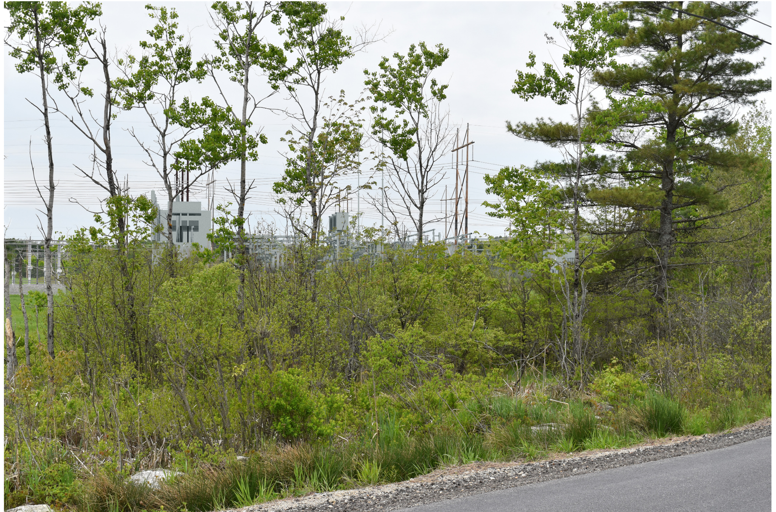
Proposed Conditions: Normal view looking from south from Fickett Road toward the proposed Fickett Road Substation and the Sections 62 & 64 Rebuild transmission lines. The visible substation components will range in height from 15' to 60' and will be silver gray in color. The closest substation components will be 450 +/- feet from Fickett Road. Other visible components will include the enclosure fence.
