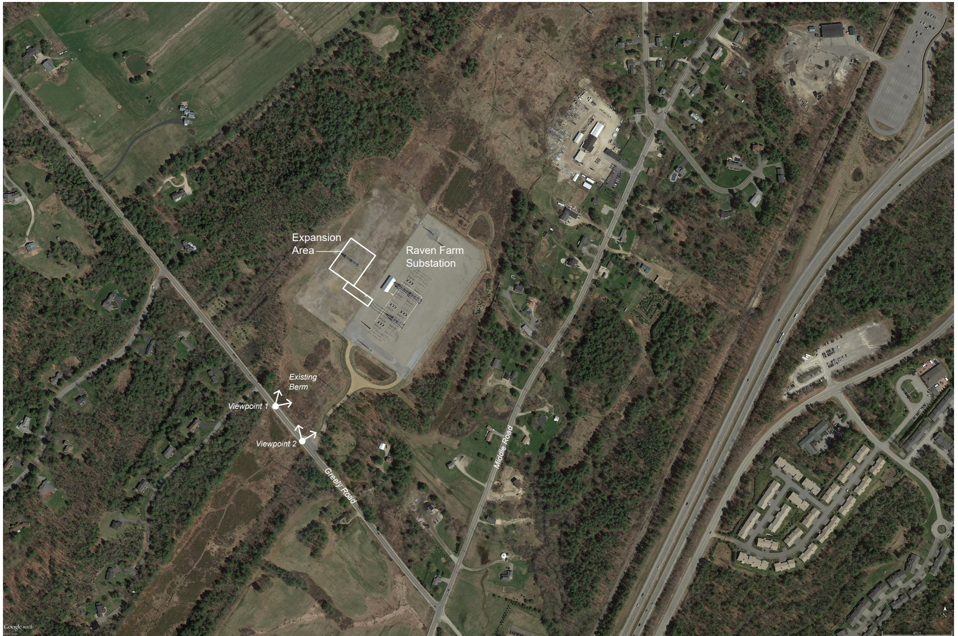
Aerial of Raven Farm Substation, Cumberland. The substation will be expanded to the northwest side in the existing gravel area. No tree removal is required.
