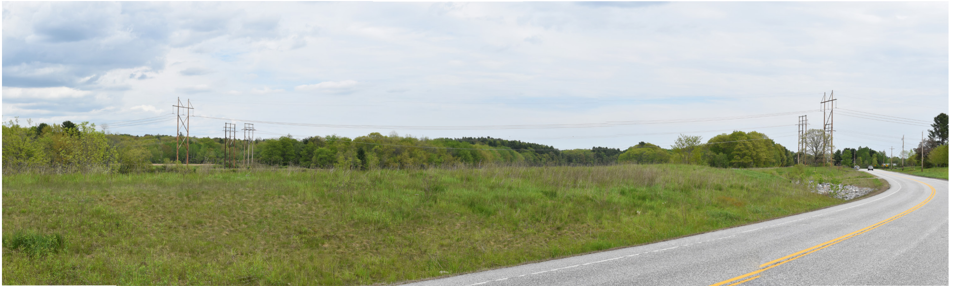
P9-10: Panoramic view looking north toward the Rebuild Sections 62 & 64 at the Androscoggin River crossing, Auburn. The two 115 kV transmission lines on H-frame structures will be rebuilt onto to single pole wooden structures. No additional tree removal is required. See Appendix D: photosimulation for view looking across the Androscoggin River.
