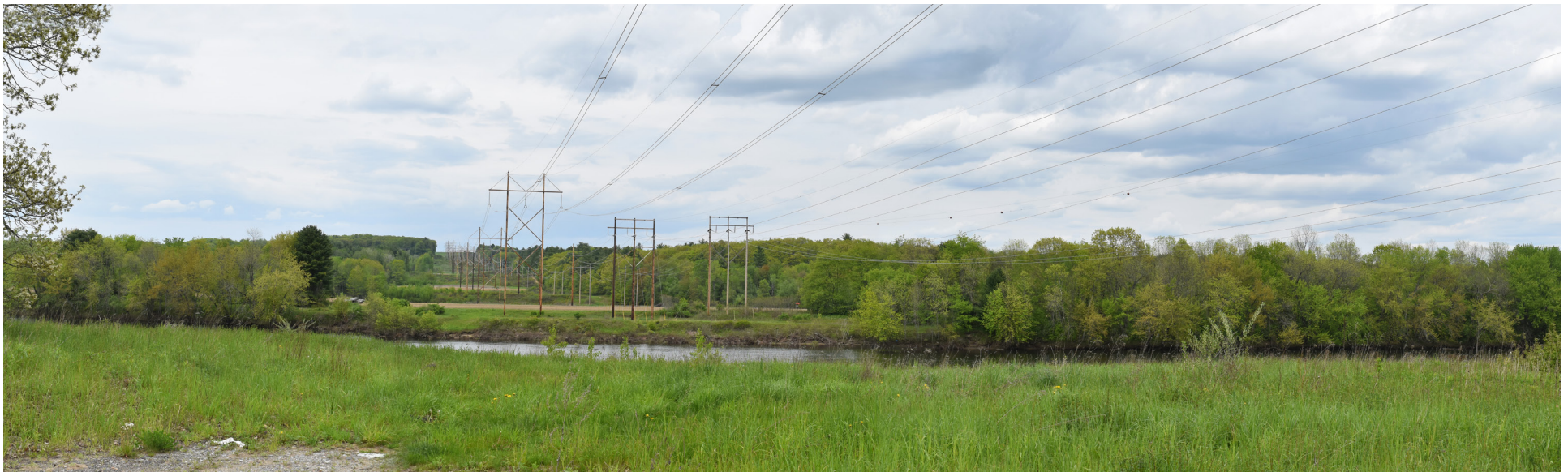
P9-11: Panoramic view looking north toward the Rebuild Sections 62 & 64 at the Androscoggin River crossing, Auburn. No additional tree removal is required. See Photosimulation in Appendix D
