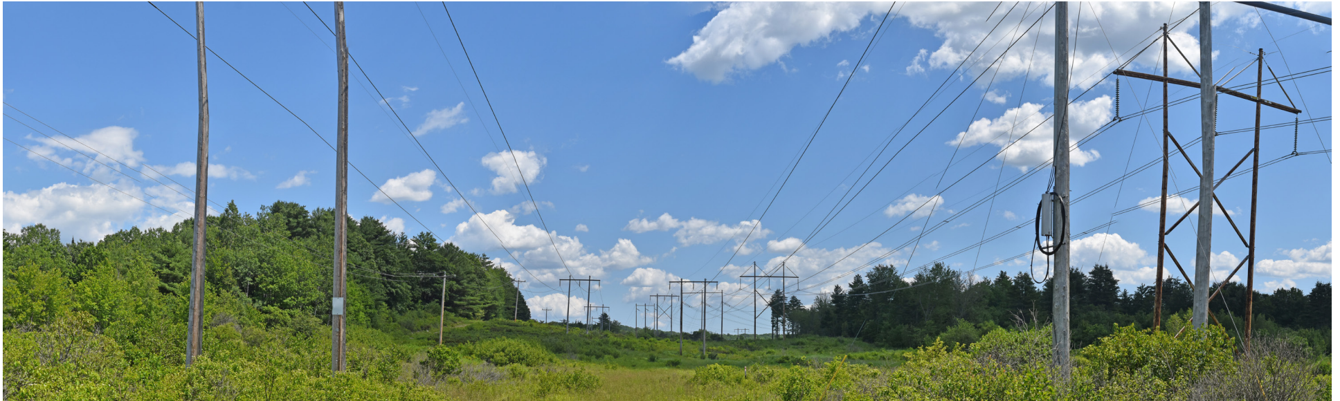
P9-3: Panoramic view looking southeast toward the Rebuild Sections 64 (one 115 kV transmission line to be rebuilt onto to single pole wooden structures) at the College Street crossing, Lewiston. No additional tree removal is required.
