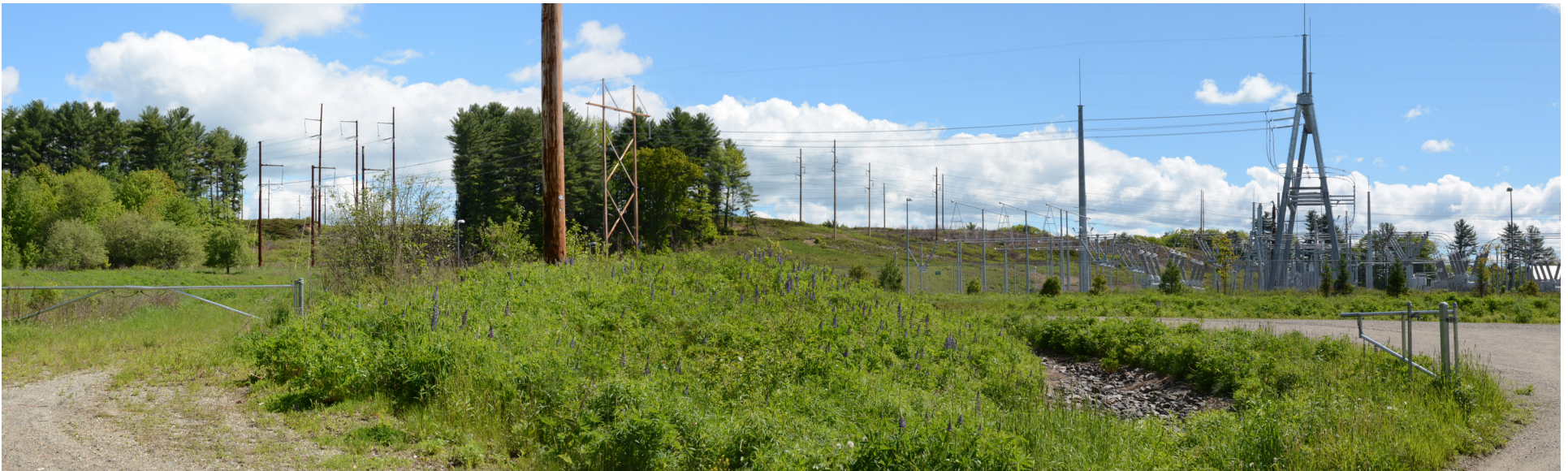
P9-2: Panoramic view looking east at the existing Larabee Road substation, existing Sections 62 & 64 to be rebuilt, and the proposed 345 kV terminal to be installed on the north side of the substation. The proposed components will be similar in height and color to existing substation components.
