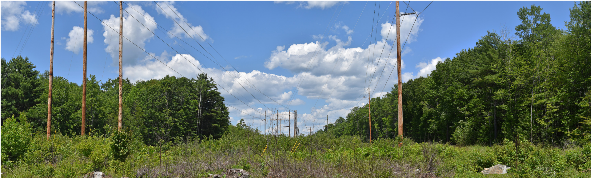
P9-1: Panoramic view looking northeast toward the existing 115 kV transmission corridor from Merrill Road, Lewiston. The existing corridor will be widened by 75' on the west side to accommodate the proposed 345 kV transmission line connection between the Merrill Road Converter Station and Larabee Substation. The Converter Station will be located 2,400 north of the road. See Photosimulation in Appendix D.
