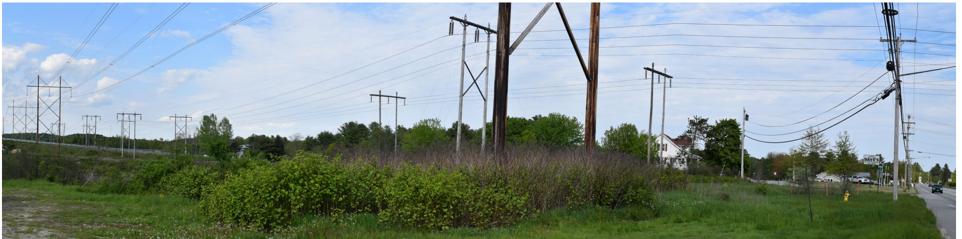
P9-9: Panoramic view looking north toward the Rebuild Sections 64 at the Route 196 crossing, Lewiston. The 115 kV transmission line on H-frame structures will be rebuilt onto to single pole wooden structures. No additional tree removal is required.
