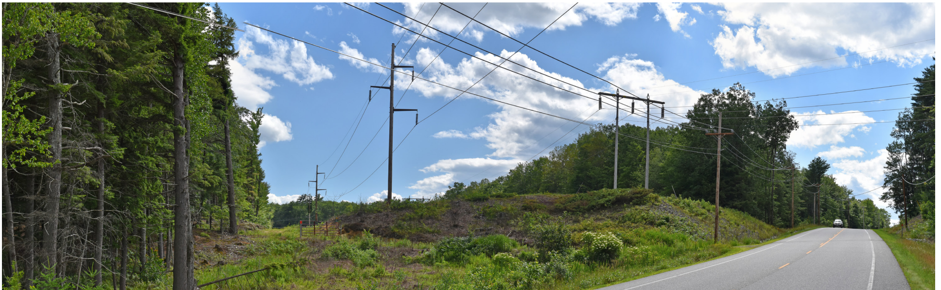
P8-12: Panoramic view looking south toward the existing 115 kV transmission corridor from the Howes Corner Road crossing (Rt. 219) in Leeds. The existing 150' wide transmission line corridor will be widened by 75' on the western side to accommodate the proposed HVDC transmission line.
