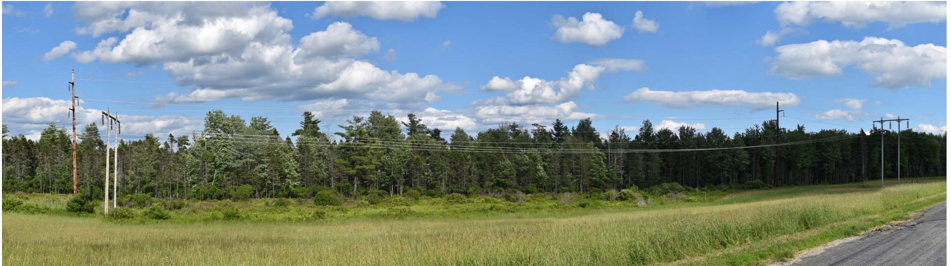
P8-13: Panoramic view looking west toward the existing 115 kV transmission corridor at the Fish Street Road crossing in Leeds. The 150' wide existing transmission line corridor will be widened by 75' on the western side to accommodate the proposed HVDC transmission line.
