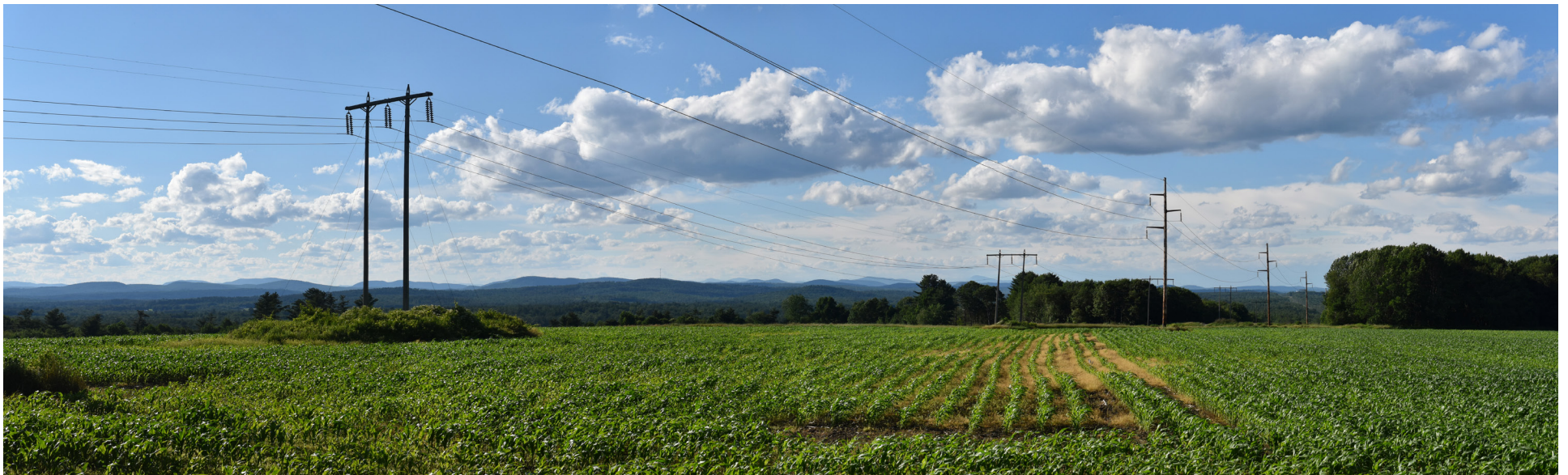
P8-16: Panoramic view looking north up the existing 115 kV transmission corridor from the Church Hill Road crossing in Leeds. The existing 150' wide transmission line corridor will be widened by 75' on the western side to accommodate the proposed HVDC transmission line.
