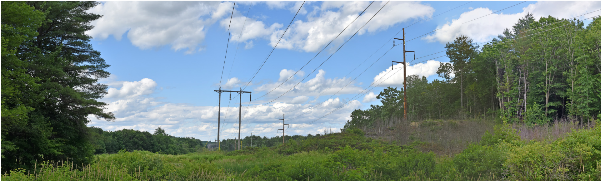
P8-11: Panoramic view looking north toward the existing 115 kV transmission corridor from the Campbell Road crossing in Leeds. The existing 150' wide transmission line corridor will be widened by 75' on the western side to accommodate the proposed HVDC transmission line.
