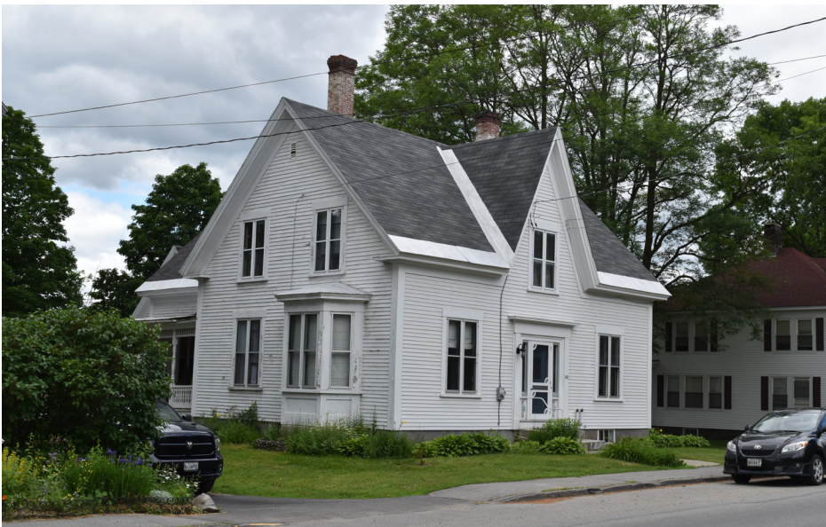
P7-6: Structure within the Farmington Historic District which is on the National Register of Historic Places. The Project will not be visible from this structure.
