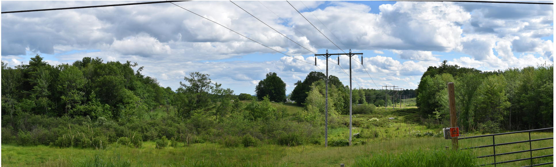
P7-17: Panoramic view looking north toward the existing 115 kV transmission corridor from the East Jay Road Crossing in Jay. The existing 150' wide transmission line corridor will be widened by 75' on the west side to accommodate the proposed HVDC transmission line.
