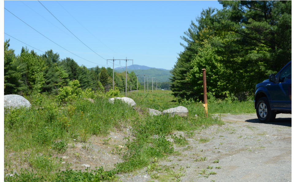
P5-6: Looking north along existing 115 kV transmission corridor at Jackson Pond Road crossing. The existing corridor will be widened by 75' on western side to accommodate the proposed HVDC transmission line.
