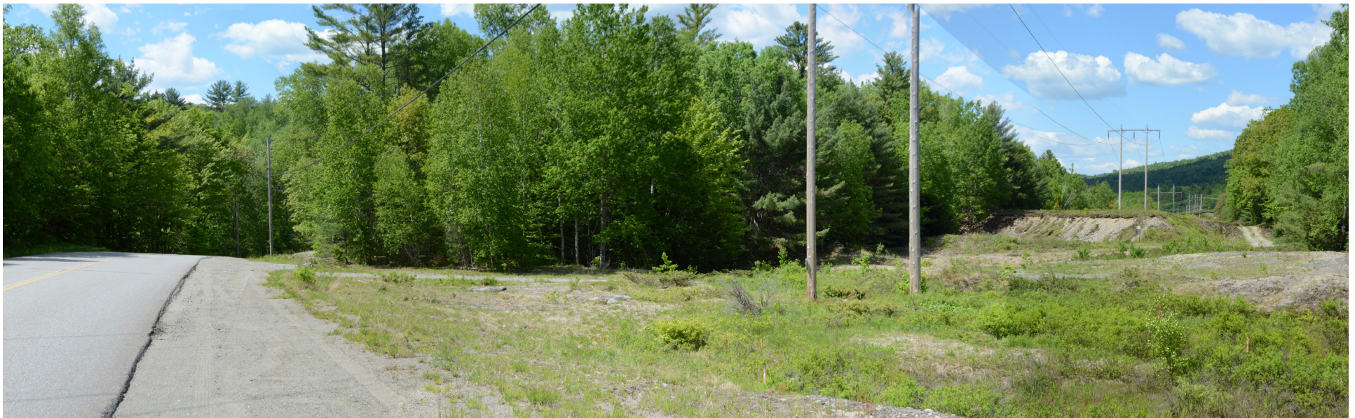
P4-16: Panoramic view looking northwest at the existing 115 kV transmission line crossing on Pleasant Ridge Road, 1 mile +/- north of the Route 16 bridge in Bingham. The proposed co-located HVDC transmission line will be located on the west side of the corridor (left in image). The corridor will be widened by 75'.
