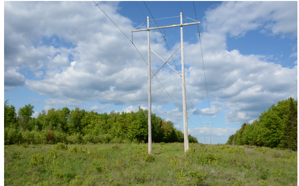
P4-10: Stream Road in Moscow near former radar station. The proposed HVDC transmission line will be located on east side of the existing 115 kV in this location.
