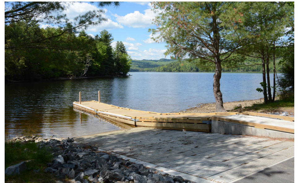
P4-14: Boat ramp at Wyman Lake Recreation Area.
