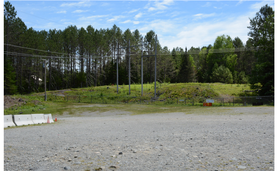
P3-6: Existing transmission lines at the parking area for Harris Dam used by rafting companies for access.
