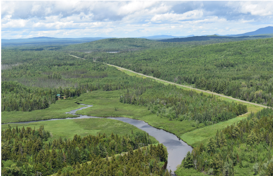
P3-26: Aerial view of the existing 115 kV transmission line crossing Moxie Stream and Indian Pond Road to Harris Dam north of Moxie Pond.
