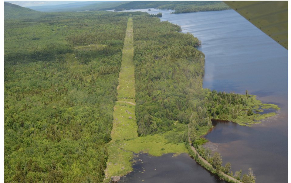
P3-27: Aerial view of the existing 115 kV transmission line on west side of Moxie Pond.
